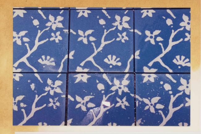
after the final grinding, the tiles are sealed with a waterproof finish.
