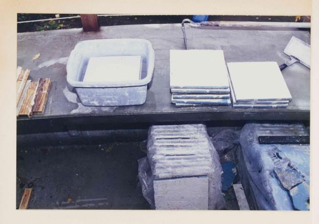
tiles are submerged in water for five minutes to ensure proper overnight curing and are covered in plastic until they can be taken to the shop for final grinding.
