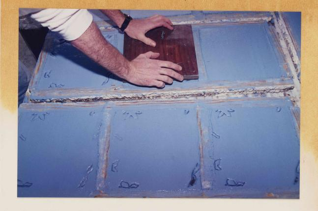
patterns are pressed into the cement. edge pattern is done first as the edges of each tile set faster than the interiors.
