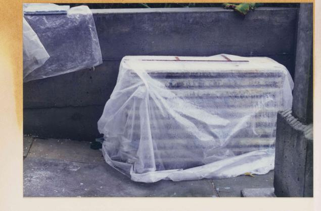
the tiles are covered and kept damp overnight to allow for setting.
