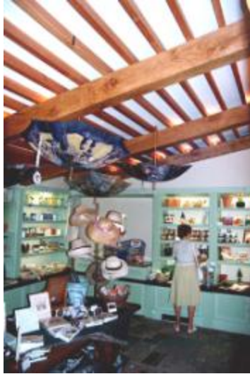
Figure 39: Gradients in the ceiling structure of the Giftshop.
