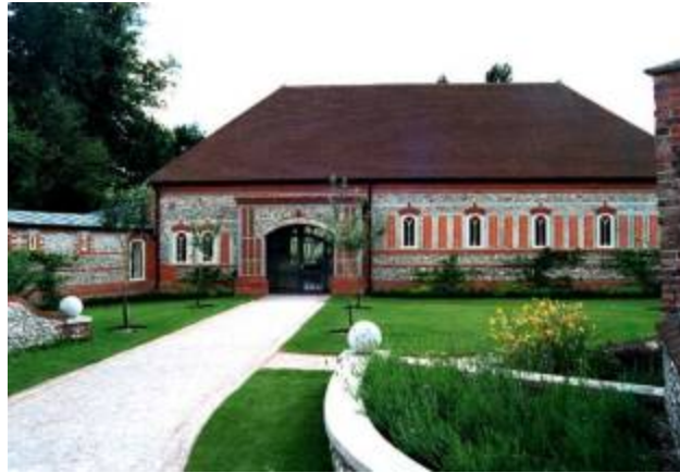
Figure 1: North facade viewed from entry path.
