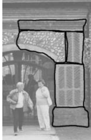
Figure 17: Right side of entry porch divided into brick base, approximately 1/5 ; lower and middle panels of brick and stone, approximately 1/2 ; upper panels of brick stone and flint, approximately 2/5 ; brick cornice, approximately 1/7 .
