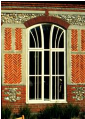
Figure 8: South Terrace facade, window of the Dining Hall
