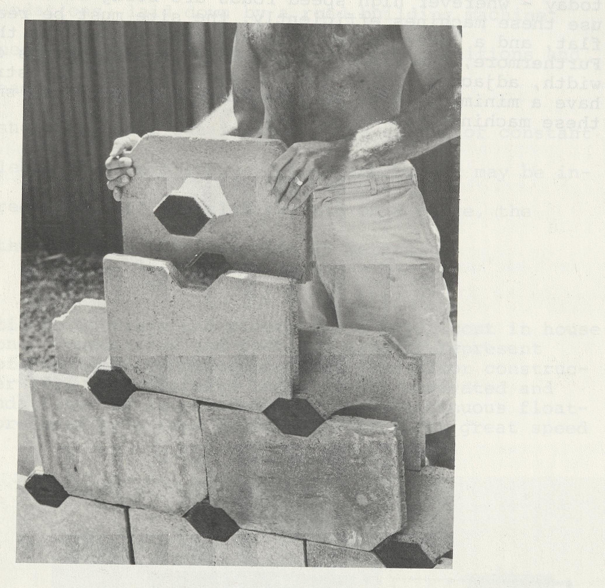
or 20 cm thick: column and corner blocks are made in special moulds. Walls and columns are reinforced with sulphur (see page 214). Plumbing lines and electrical conduits run through the cavity.
