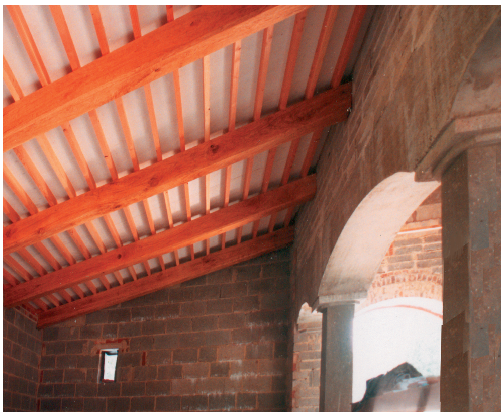
The emerging order of the West Dean structure seen in one of its arched cross-walls
