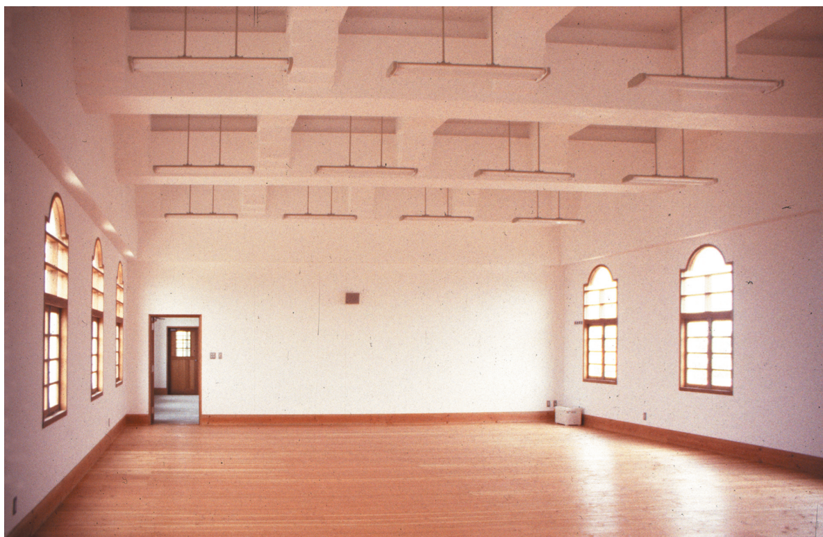
Interior of Northwest college building, showing the simplicity of form, and the mat of horizontal beams acting to transfer horizontal forces through a moment-resisting diaphragm formed by the beams
