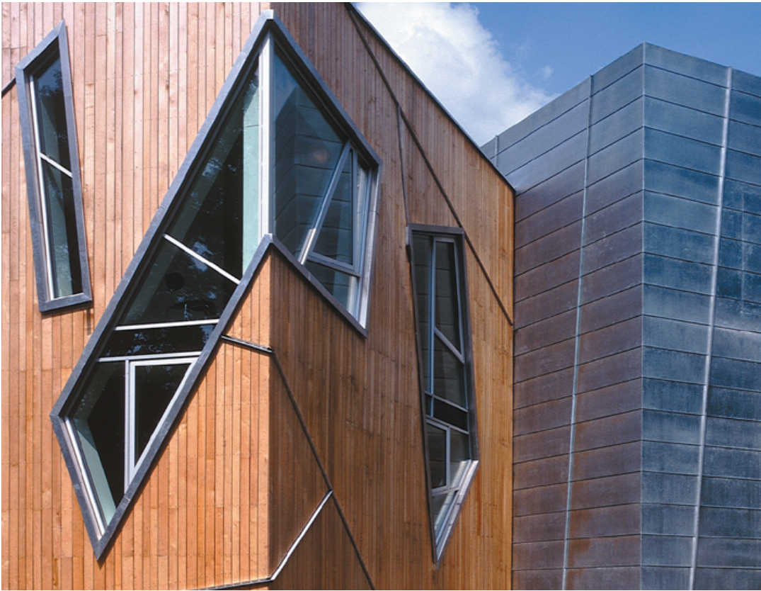
Twentieth-century form language: The schemata here are not useful for creating living structure. Daniel Libeskind, Felix Nussbaum Museum, Osnabrück
