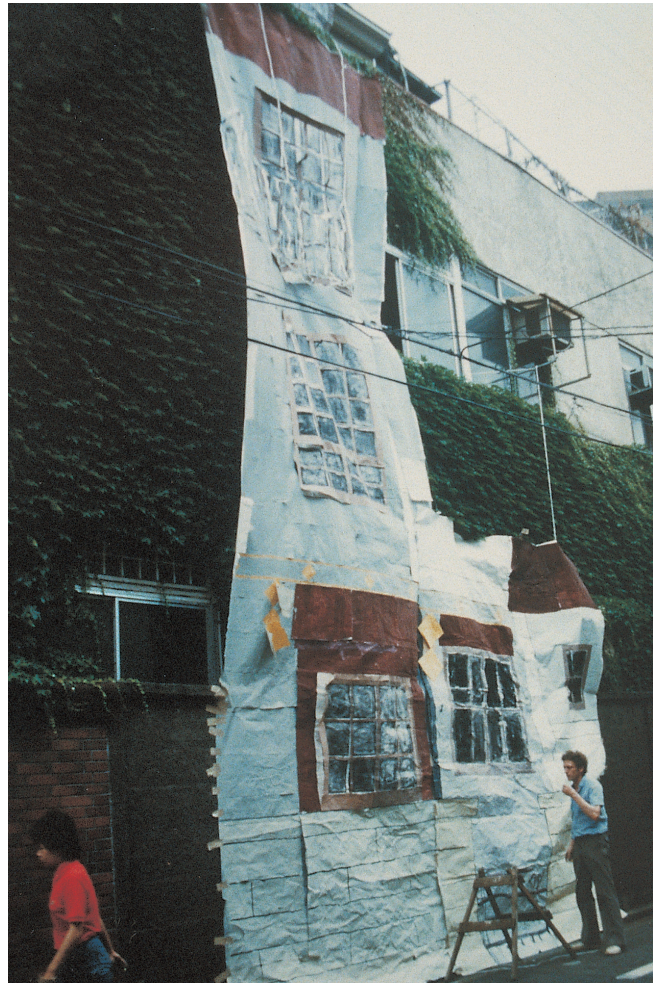
Emoto Apartment Building, Komagome, Tokyo, Christopher Alexander, Hajo Neis, Ingrid King, 1987. This full-size three-story mockup in Tokyo, done in paper to study the effect of the elevation design and materials on the street at actual size, was done to make sure that the street was helped by the building. Mockup by Hajo Neis.
