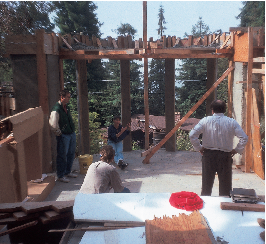
Settling positions of columns, to form the bays and window openings of the living room bay window
