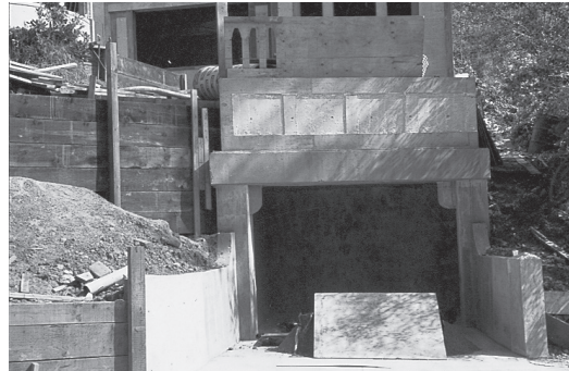
Formwork on the massive concrete brackets which frame the garage
