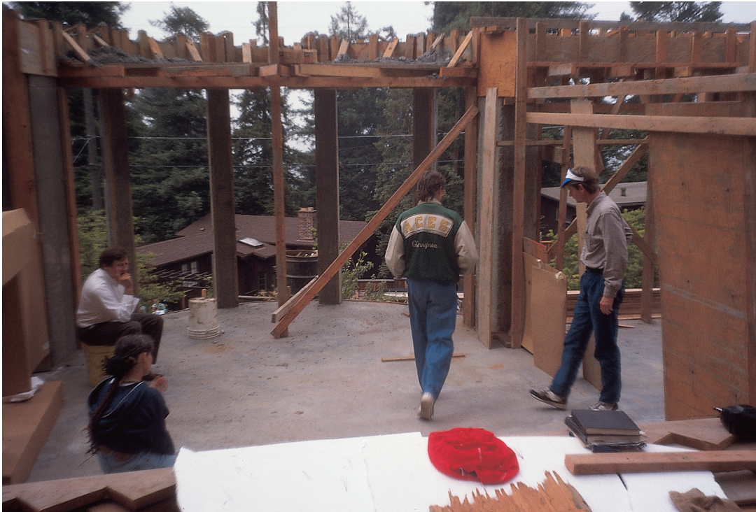
Walking into the room, testing the position of the door, and trying to find out if the positive space of the bay window is large enough, when the door is in a certain position. We moved this door several times, and finally tuned it to within about two inches to get its best position.
