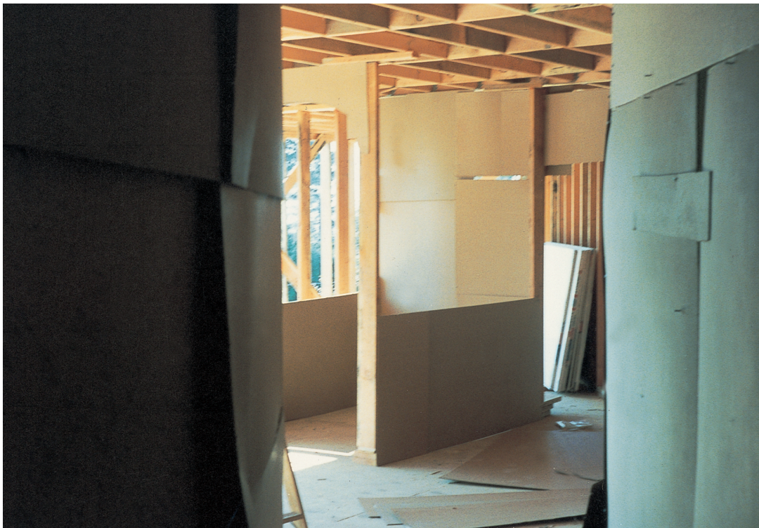
The upstairs after rough framing, and before new decisions were made. The cardboard walls and mocked-up partitions showed us clearly just how bad it was.
