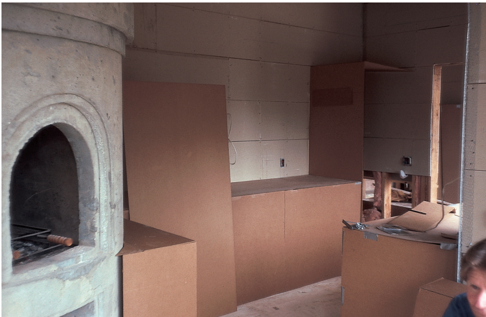
The kitchen mocked up in its entirety in cardboard, so we could see just how to make the kitchen fireplace. The idea of a cylinder had already occurred to me from seeing the room shape and recognizing its two lines of sight. Now we had to make the cylinder work, and to do that we had to have the full three-dimensional configuration, as it was going to be. We had to make many many versions before it all sat right.
