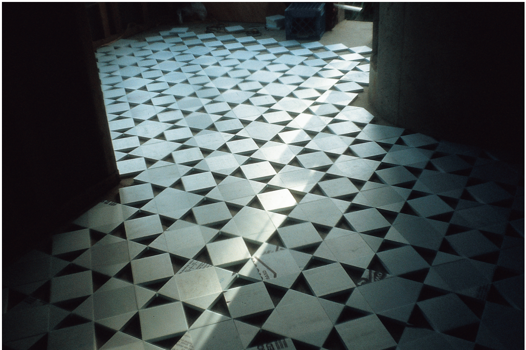
Styrofoam forms from the making of the kitchen floor, in preparation for the first colored terrazzo to be poured into the voids between the pieces of styrofoam (white)
