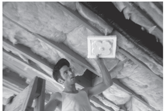
Trying the size and weight of one of the versions of the rosettes to go in the middle of the ceiling panels
