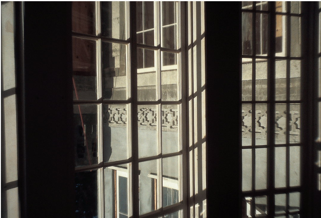
Close-up of living room windows after installation
