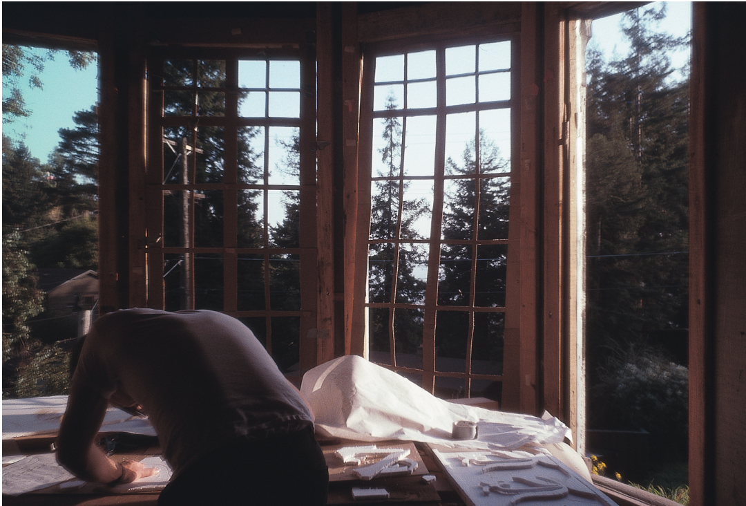
Cardboard mockup to test the size and distribution of glazing bars in the windows of the living room. This was about the fifth version: it took that long to get it just right.
