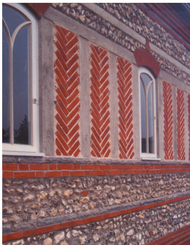
The north wall: windows, herringbone-brick panels, flint.
