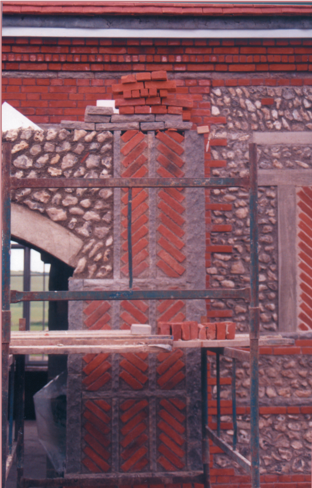
The Entrance Porch, under construction, West Dean Visitor's Centre, 1995
