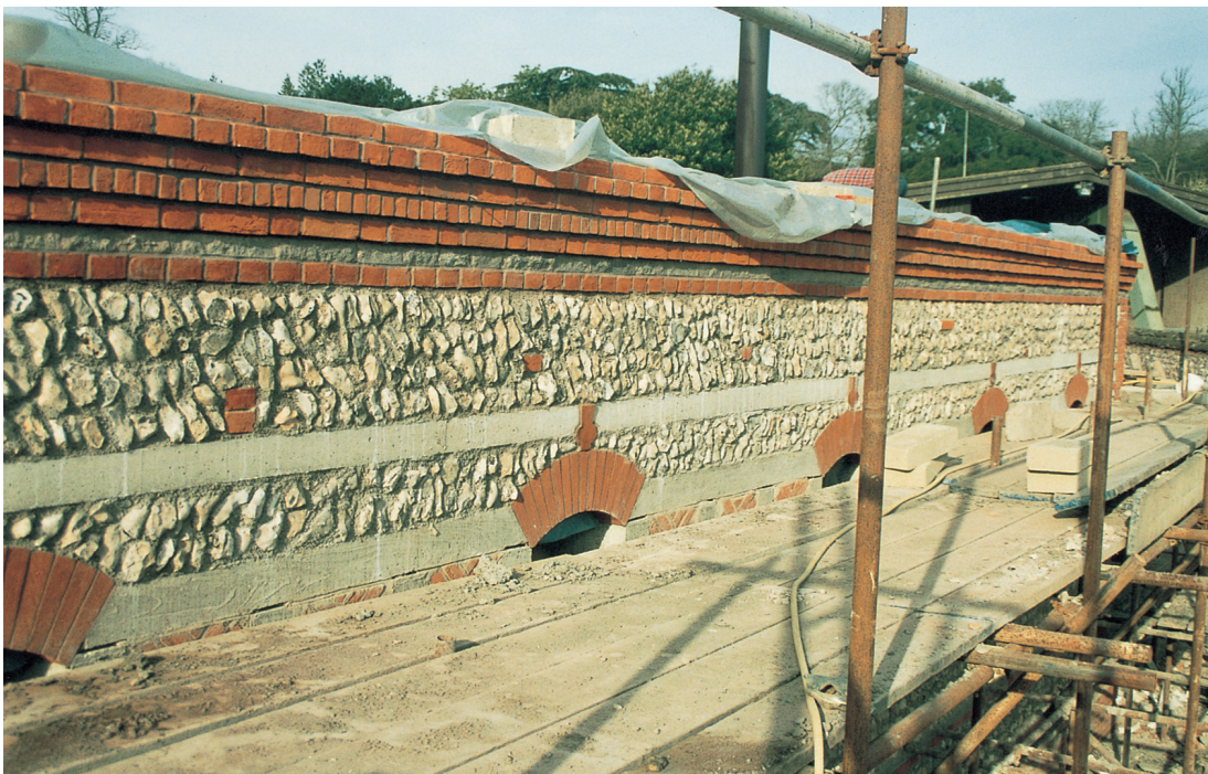
Here we see the handling of brick, headers, flint, and stone, that we worked out, course by course, to give the cornice at the top of the north wall a true I-like character. It took many experiments, and every course had to be placed by eye, in mock-ups, to make the whole thing come out right.
