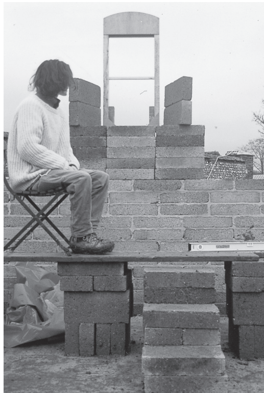
Getting a first fix on the position, size, width, and splay of the large southern windows. By placing chairs, and sitting down as if one were in the finished building, it was possible to give the window opening the being-character that emerges most naturally from this situation (middle left). Testing the size, width, position, and extent of the tiny stairs that come from the gallery into the main dining room—looking, once again, for the exact proportion and size which would make these stairs connect us with the I (lower left). Sitting in a mockup of the upper gallery, and testing the splay and depth of the window reveals, to get their shape and character just right (bottom right).
