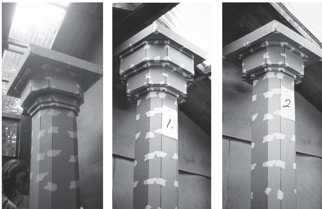
While trying to work out the column capital with the most being-quality, we made a series of full-size cardboard mock-ups, and looked at them in the space where they were going to be built. In the end, all of these shown here were rejected, and the much simpler shape shown on page 128 was chosen as the one which had deep life most profoundly.
