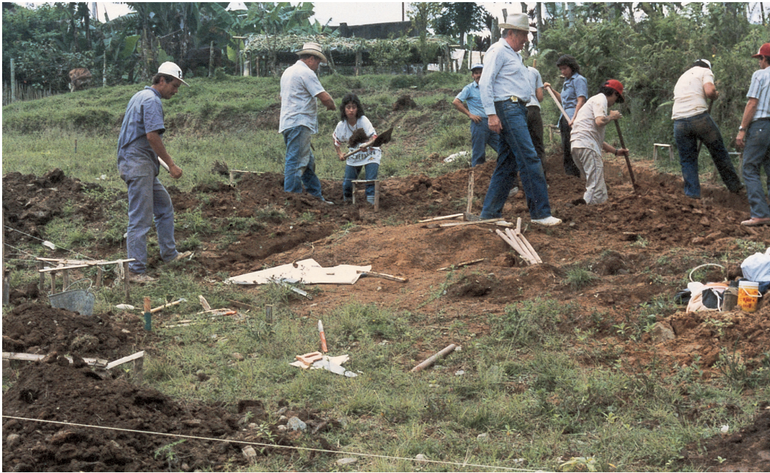
Families working on site
