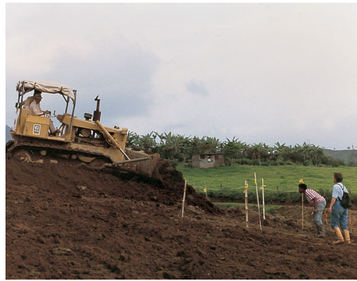
Placing stakes to define a house volume
