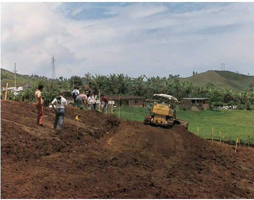
Preparing a lot for staking out
