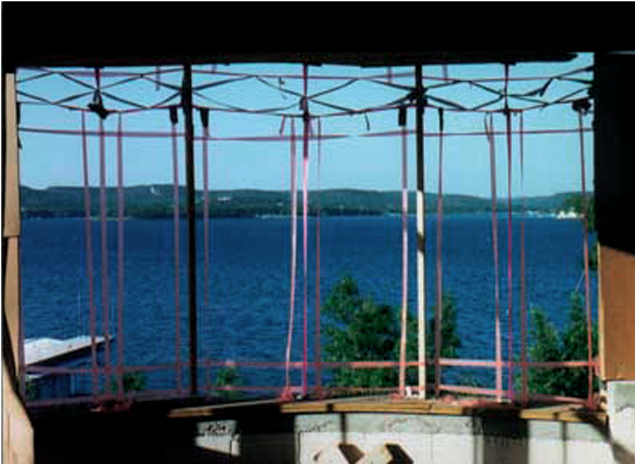
Mockup we did to get the pattern of glazing bars for the windows in the dining room. We adjusted the tapes you see in this photograph, until they formed a beautiful pattern and enhanced the lake. Then we had the windows built. Christopher Alexander, Randy Schmidt, 1996.
