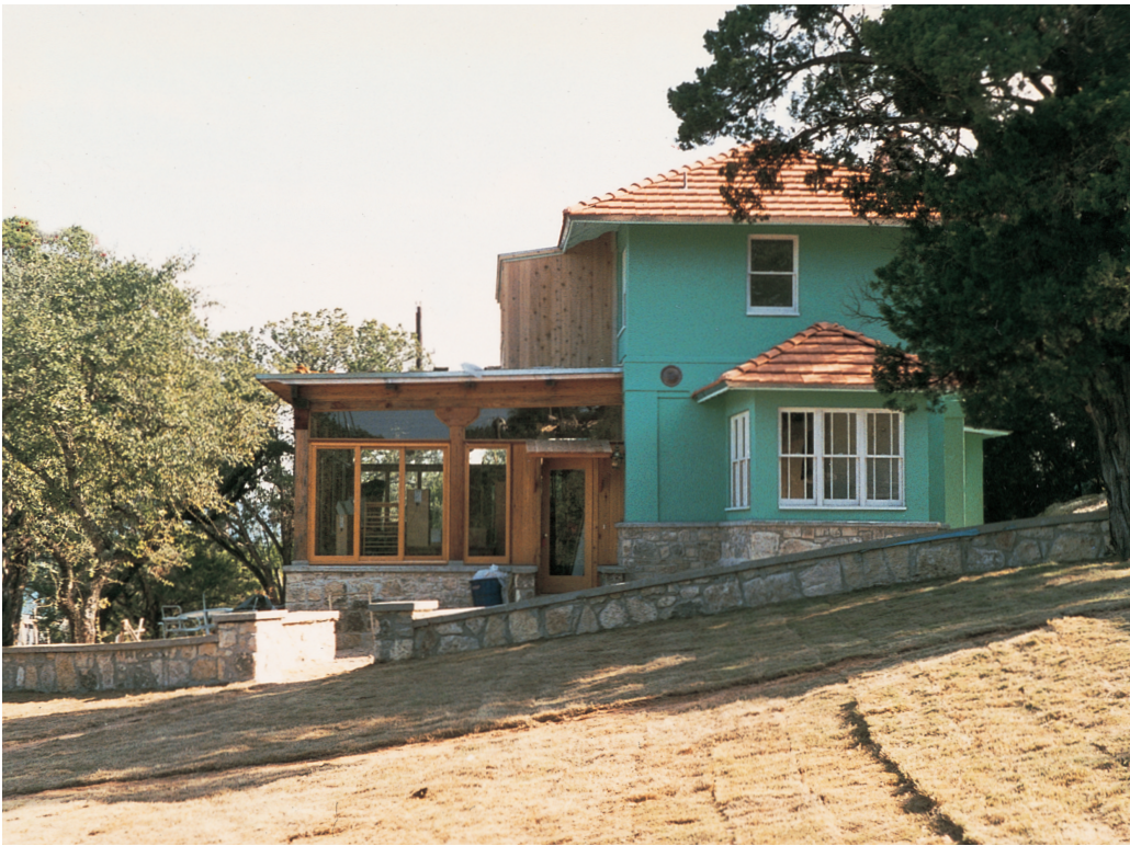
Heisey house, Back of the Moon, Austin, Texas. Christopher Alexander, Saul Pichardo, Randy Schmidt, 1996.
