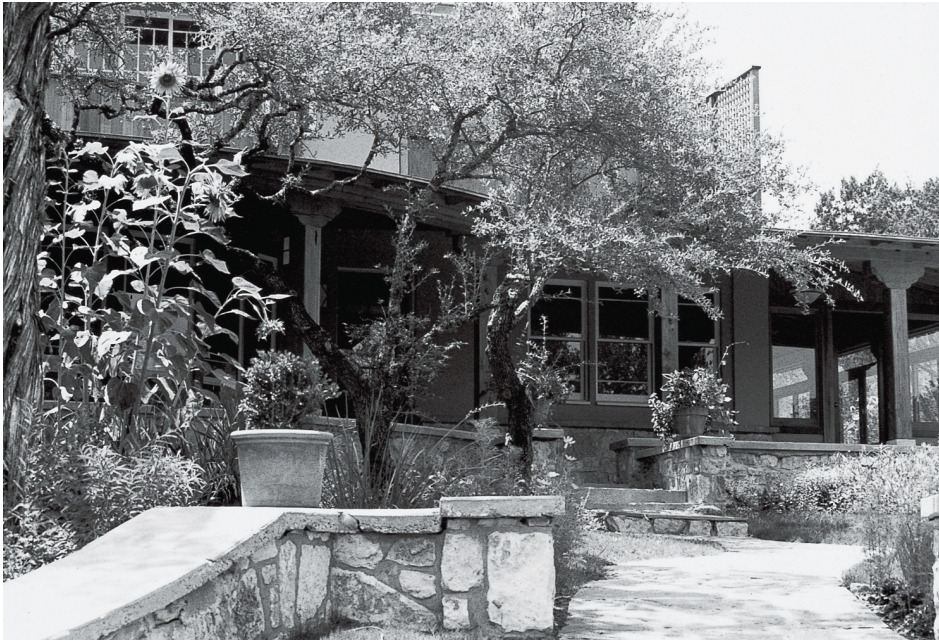
Steps leading up to the entrance of the Goddu house.
