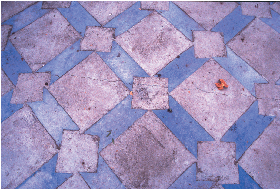
Ornamented concrete slab in the Fresno Farmer's Market, made by precasting 1/2 inch thick light blue fishtails, then dropping them into the slab while the slab was wet and still being worked, floated and troweled. Christopher Alexander et al., 1984.
