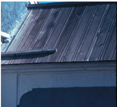
The Russian roof on the Martinez building, California.
