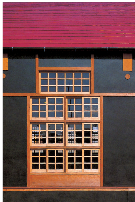
Orange-painted steel bracket plates on the Gymnasium.
