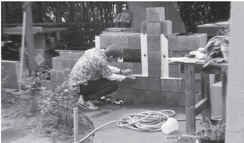
Massive stones being checked for the Hodgson house, California. The stones are cast concrete. Each one has a dark surface; the surface is cast, then washed with a light water wash. Inset, or inlaid next to the stone, is a chase to receive a fine line of white marble.
