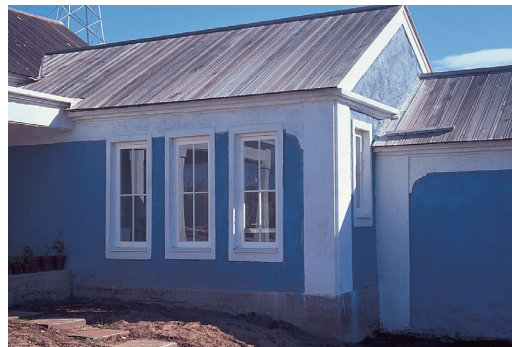
Detail of the outer layer of lapped boards in the Russian roof.
