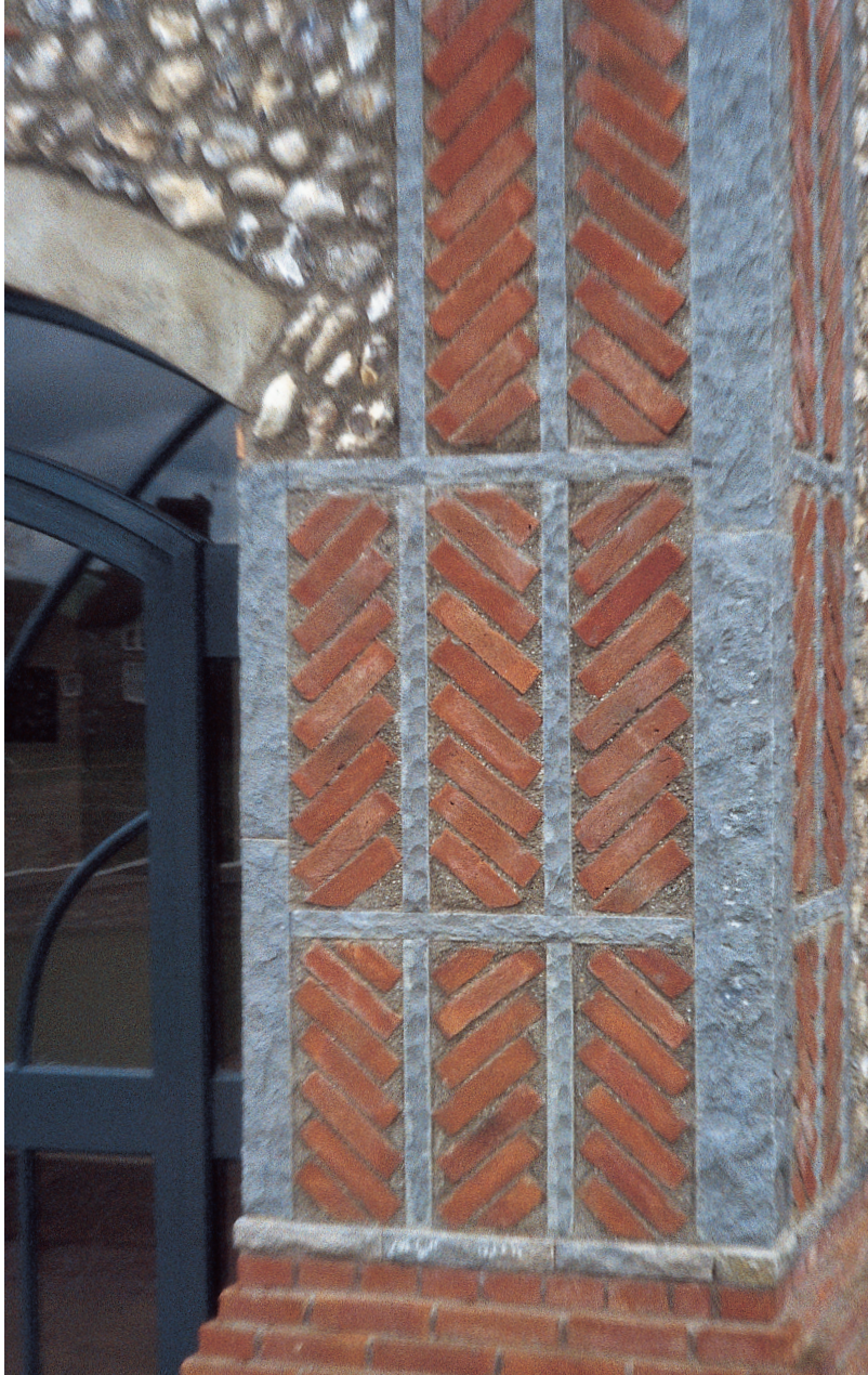
Stone and brickwork on the entrance porch of West Dean: the stones are cut in thin lines, and together with the panels and herringbone bricks, have been chosen to make the porch wall of STRONG CENTERS with GRADIENTS, ALTERNATING REPETITION, STRONG CENTERS, LOCAL SYMMETRIES, CONTRAST.
