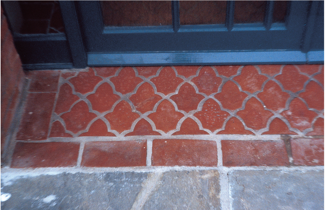
Floor tiles, made to our design, forming centers over the floor surface of the West Dean building.
