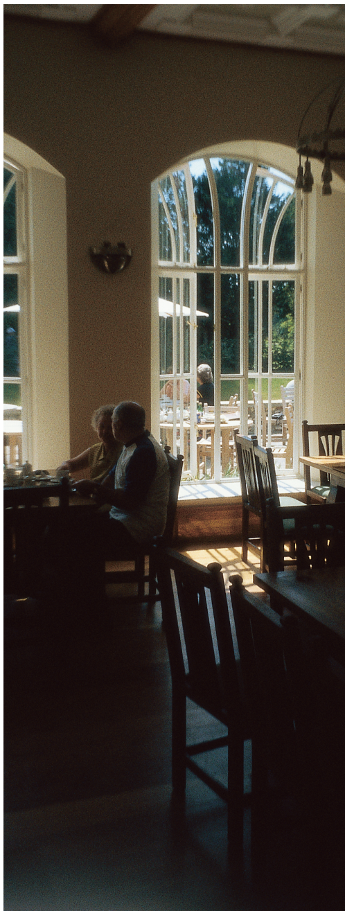
Curved window with specially made arched head and curved glazing bars. Christopher Alexander and Derek Bonner, 1995
