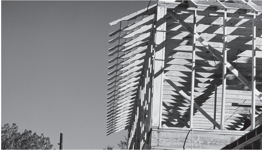
Shaped rafter tails to form a roof edge and eave. The eave is more complex, and made a better center, by the shape of the tails. Back of the Moon project, Texas.
