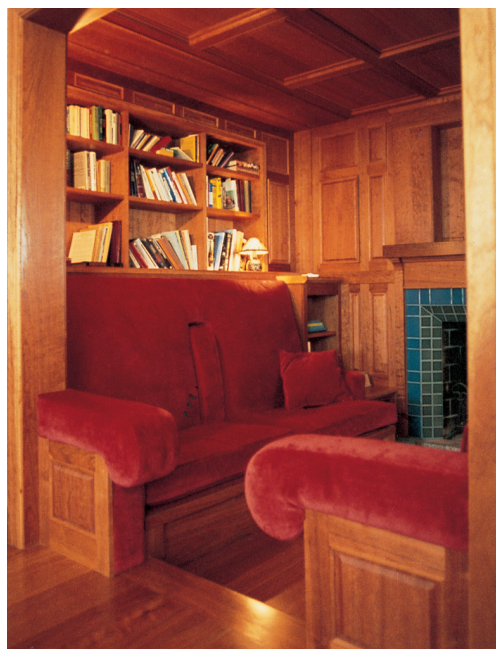
A wood-paneled fireplace nook, where upholstery is built into the hardwood arms of the physical structure. Sullivan house, Christopher Alexander and David Soffa, 1995.
