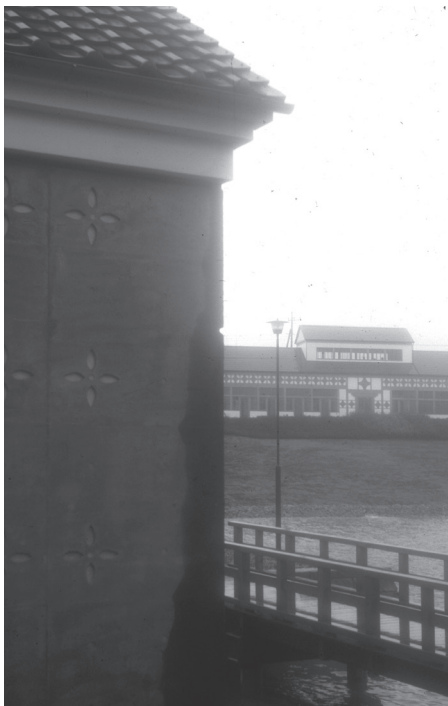
Example of the eave from one of the classrooms at Eishin.
