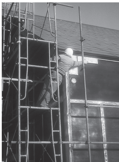
Judging the eave detail, during construction. Gymnasium, Eishin Campus, Tokyo.
