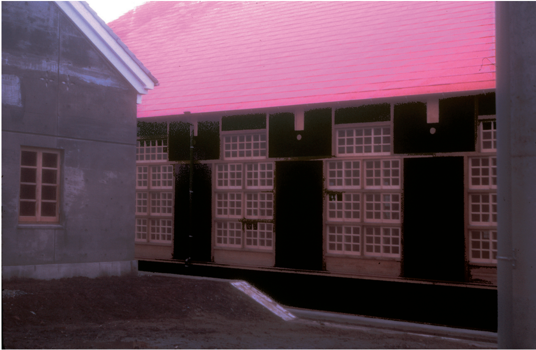
The eave, the end of the truss, plus the windows of the Gymnasium on the Eishin Campus shows an example of such a "whole." The eave was being tested and perfected at the same time as the unusually shaped windows in the long wall. It is the cooperation of these elements together, working together to form a harmonious whole, which reflects a holistic operational step of the kind described in the text.
