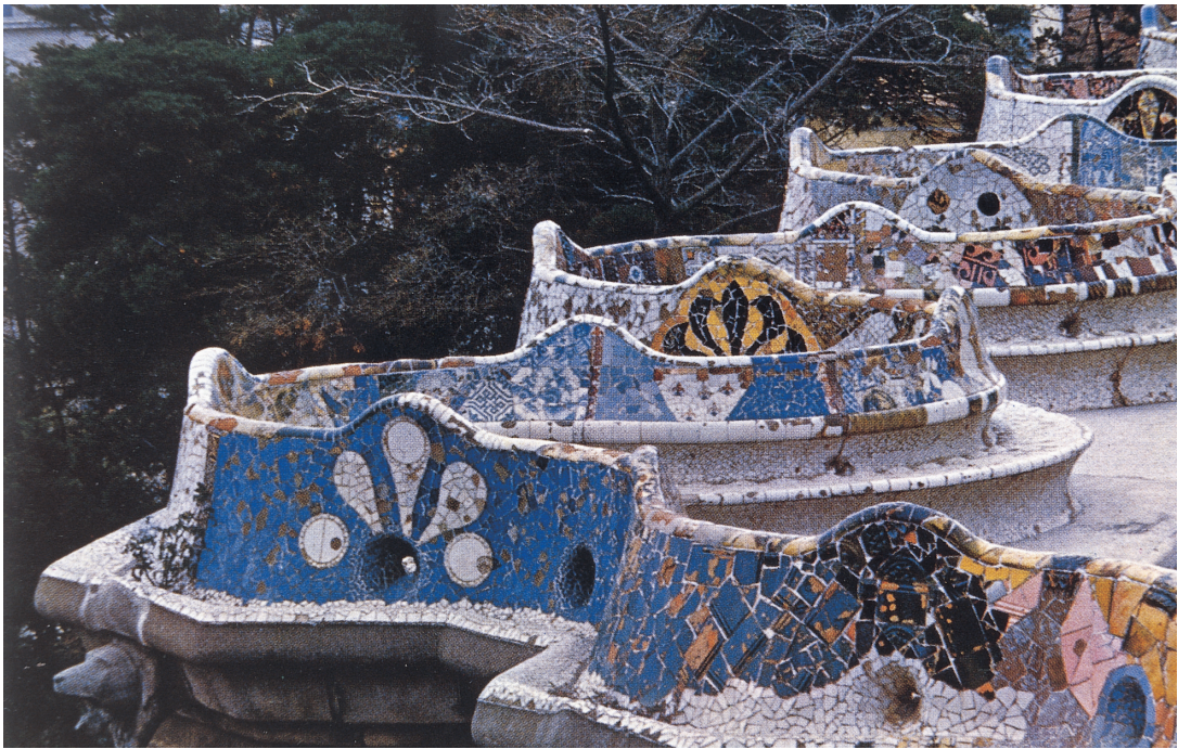
The plasterwork minutely adapted, the broken tiles then adapted to the curves of the plasterwork. Antonio Gaudi, Parc Guell, Barcelona, c. 1915.
