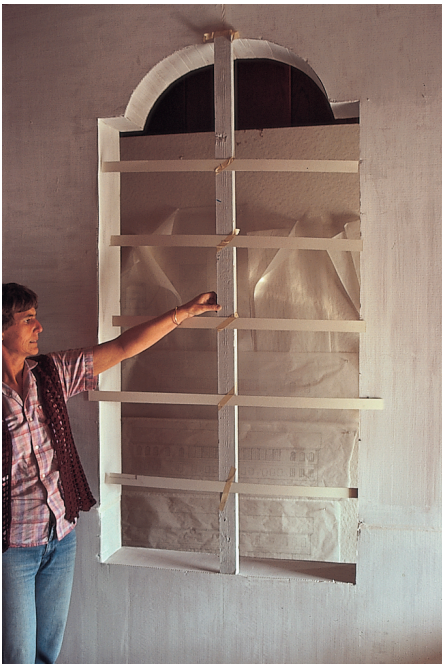
Mockup for a window. This fully formed cardboard model, made in our shops in California, once detailed to my satisfaction as sufficiently profound in feeling, was then translated into carpentry by our carpenters in Japan.
