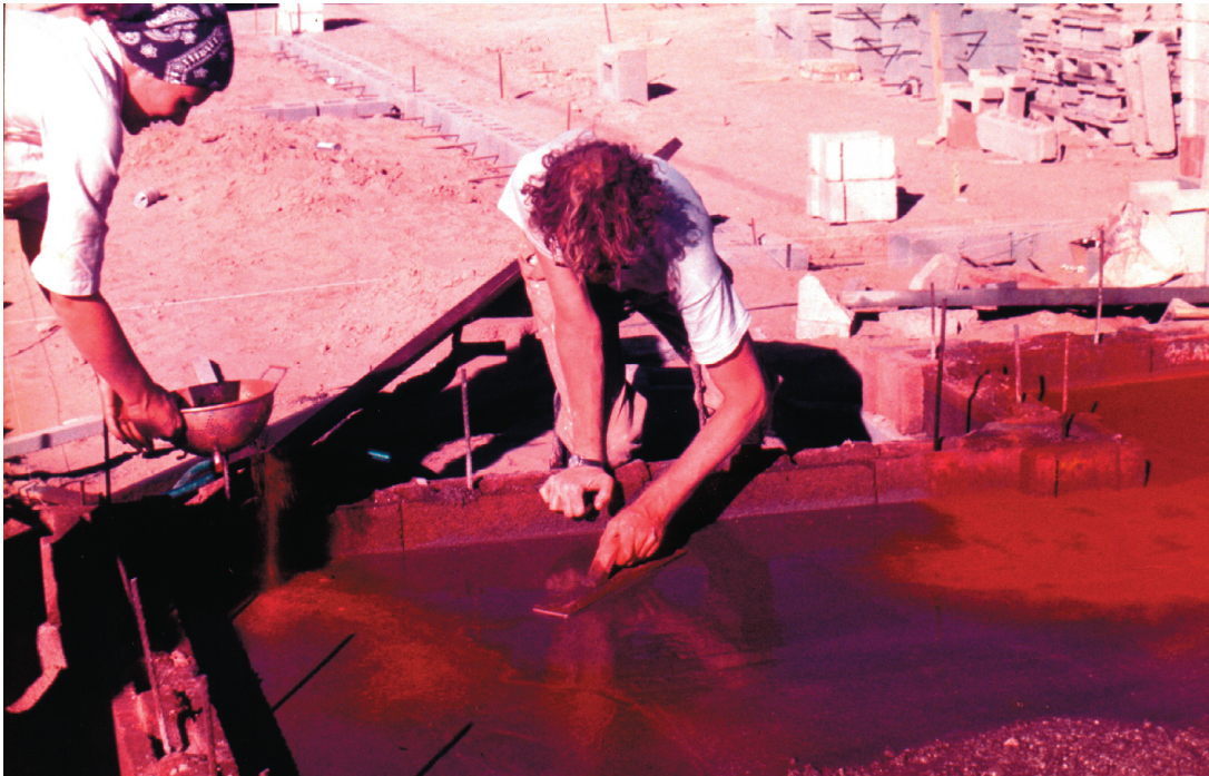
Hand troweled slab, Mexicali. The red oxide was mixed with sand and scattered on the wet slab through a sieve, then troweled hard.
