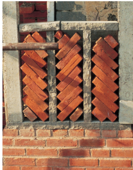
Making a mockup for an entrance porch with brick plinth, stone verticals, red herringbone inserts.
