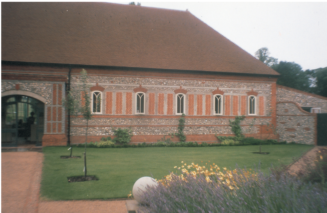
The corner on the right is differentiated by the presence of the window.
