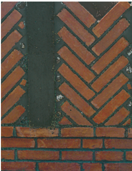
Making a mockup for an entrance porch with brick plinth, stone verticals, red herringbone inserts.
