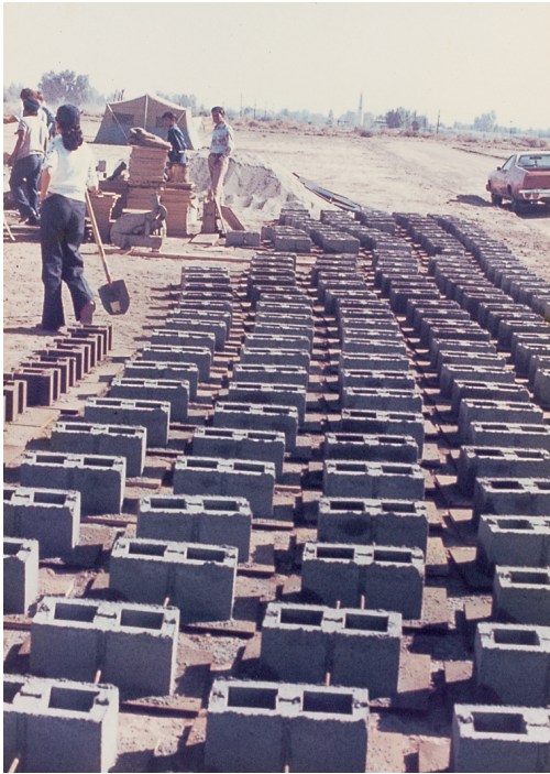
Left: Special blocks for the Mexicali project, as we manufactured them. The design of our cylindrical blocks allowed round columns to be made, both beautiful in design and easy and cheap to make, thus allowing “making” to go on rather easily. Right: Two of my apprentices designing, and making the entrance arch to the Mexicali housing. Design and construction are more or less inseparable.
