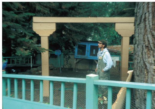
Cardboard mockups in our Berkeley yard, 1500 miles from the building site where our crews were working. On the left, our first try, a capital that is too shallow, not substantial enough to work with the beam. On the right, our second try, a capital that is too deep, too fat.
