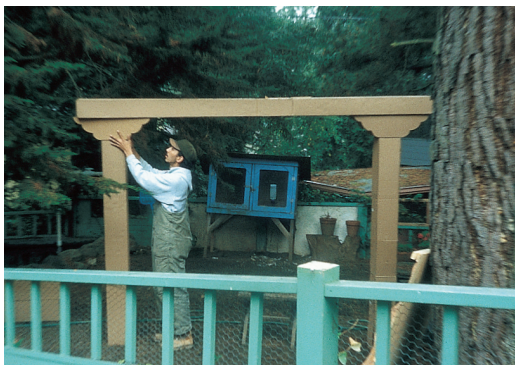
Cardboard mockups in our Berkeley yard, 1500 miles from the building site where our crews were working. On the left, our first try, a capital that is too shallow, not substantial enough to work with the beam. On the right, our second try, a capital that is too deep, too fat.
