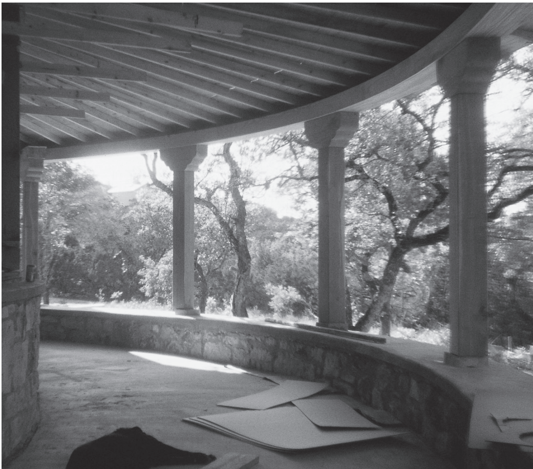
The shape of the finished column capitals, showing the result of work in the Berkeley yard, translated into actual construction. Here we see the powerful impact of these carefully-shaped columns and capitals on the space of the porch of the Goddu house, Austin, Texas. In this picture the house was still under construction.
