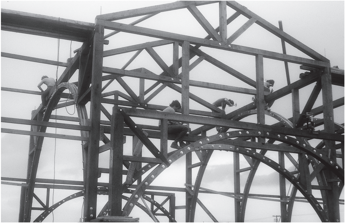
Timber framing process with erection of prefabricated frames, in the Farmer's Market, Fresno, California. Christopher Alexander and Carl Lindberg, 1986.
