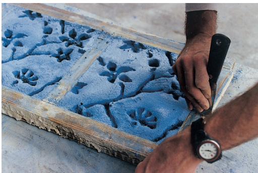
Left: Blue terrazzo in place, white not yet troweled in. Right: Cleaning a tile. The completed floor is shown on page 585.
