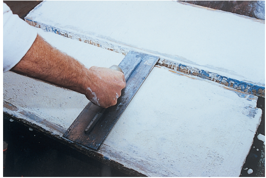
Troweling in the white terrazzo after the blue has hardened
