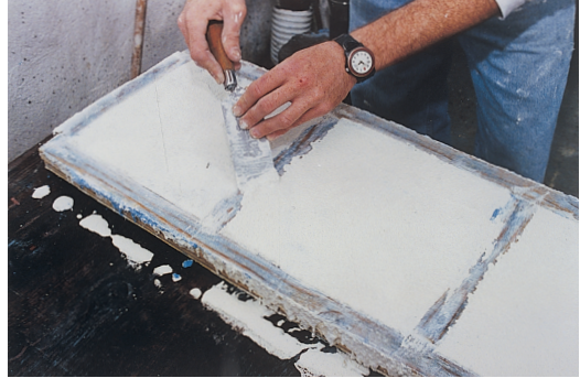
Cleaning off the excess white terrazzo
