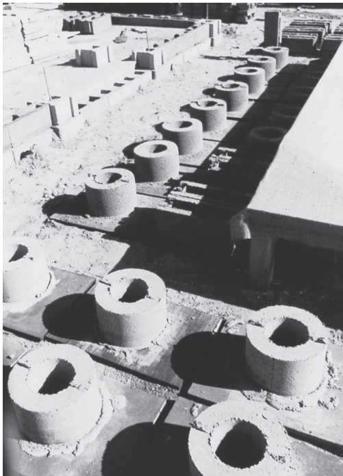
Left: Special blocks for the Mexicali project as we manufactured them. The design of these cylindrical blocks allowed round columns to be made, both beautiful in design and easy and cheap to make, thus allowing "making" to go on rather easily. Right: Two of the special molds we made for fabricating blocks. In the illustration on page 551, the protruding reinforcing steel is clearly visible coming out of the side of each foundation block.
