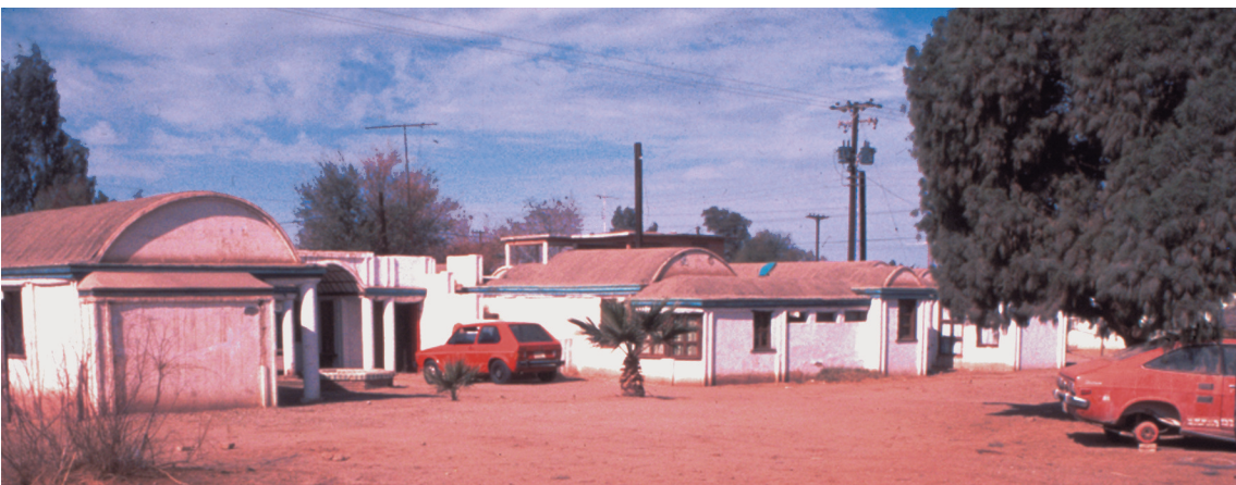
Variety of houses as a natural part of the community of houses built using this technique of unfolding. Without introducing any additional construction cost, each house turns out unique and different according to its situation.
