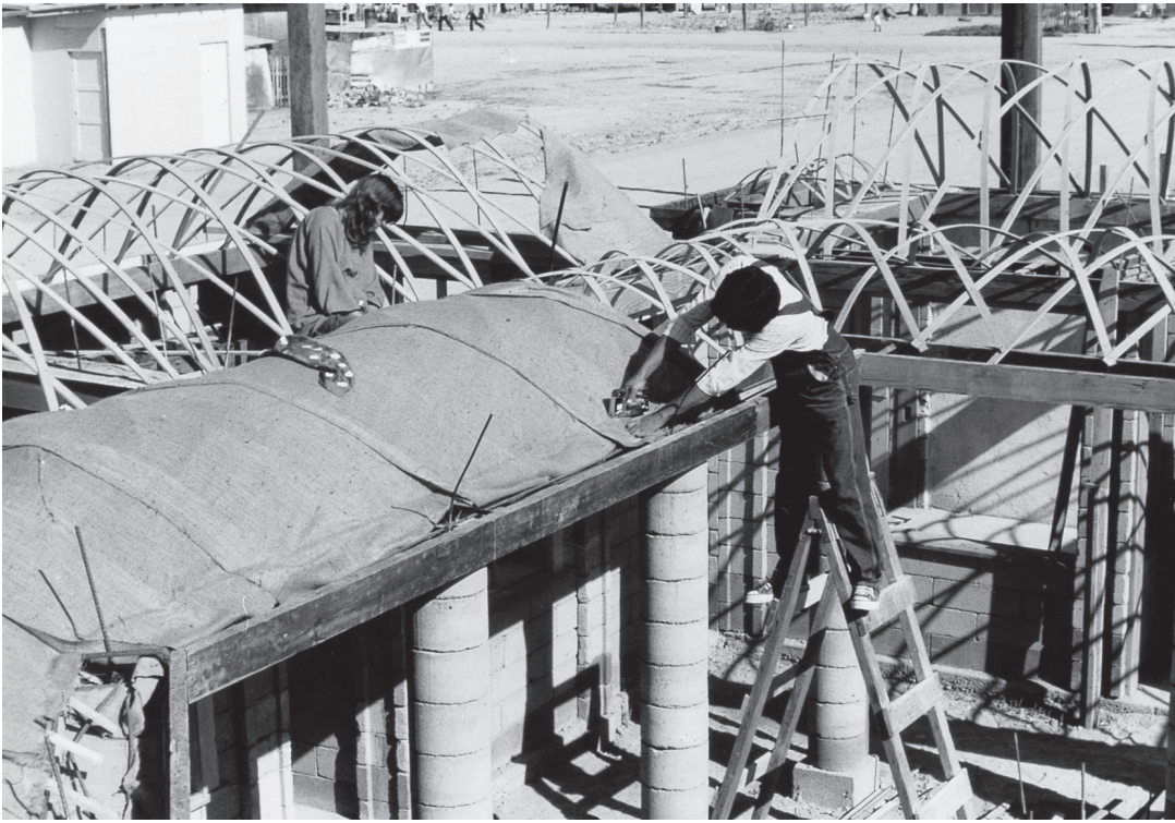
Stapling the burlap over the woven baskets once the baskets are complete.
