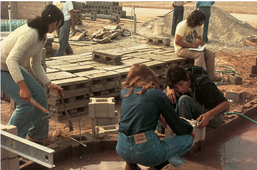
Our manufacture of special interlocking earth-cement blocks designed so they could be placed in a way that allows unfolding to proceed smoothly and without backtracking.
