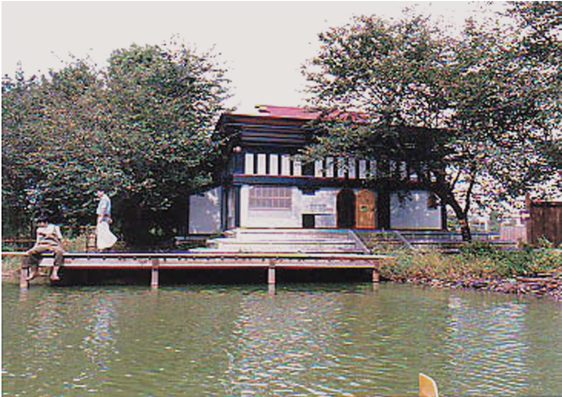
The new clubhouse with a structure of large members showing the beauty which this formation of members achieves. Christopher Alexander, Randy Schmidt, Masaya Okada, Miyoko Tsutsui, completed 2002.
