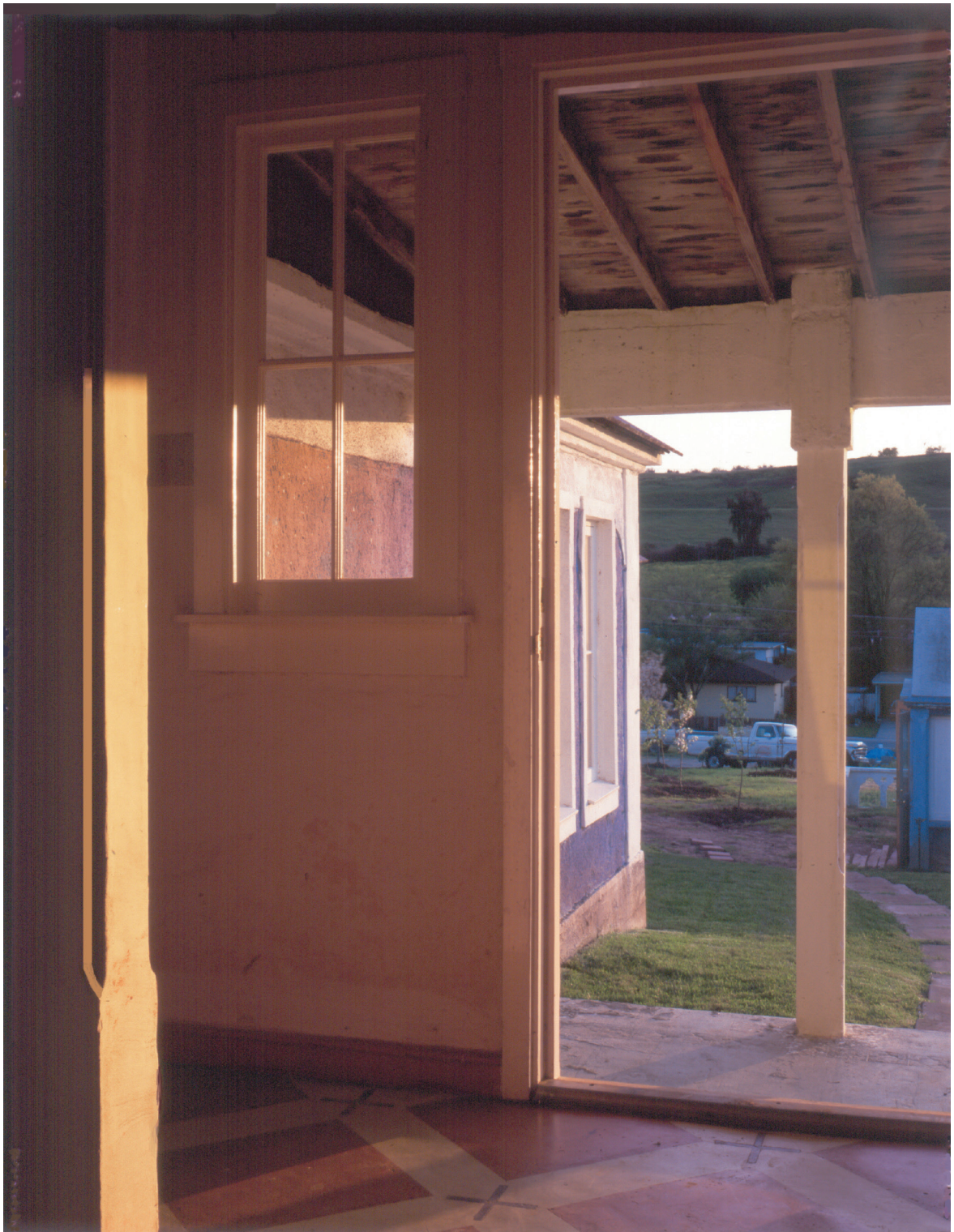
Evening: a view from the porch of the Martinez house. The concrete walls, beams, and columns are all made with ultra-low-cost formwork, shot by the new techniques which are described in the text. We built this house (which later became one of our offices) over a period of time, and various CES staff at different times worked on it with me at different times, including Harissos Tsiringas, David Dacus, Gary Black, Olasheni Agbabiaka, Jonathan Fefferman, Carl Lindberg, Eleni Coromvli, Seth Wachtel.
