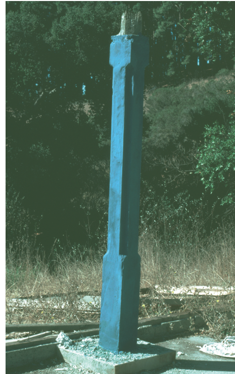
A recently invented, process-based technique. Left: Guidework for a column that is to be shot in gunite. Upper right: The jig I made so that I could cut compound curves on a two-by-two to build the corners of the form. This curve, cut off the plane of the diagonal, allows a flare to be created, making an elegant (and cheap) transition from the column shaft, to the capital and base (the finished shape that comes out is visible in the lower picture). Lower right: One of the first experimental columns, showing the result of shooting gunite into such an open form. The flare created by the cut two-by-two is visible on the corner of the column, where shaft meets base. In the picture on page 523, you may see columns of this kind in one of our building projects. Christopher Alexander, 1979.
