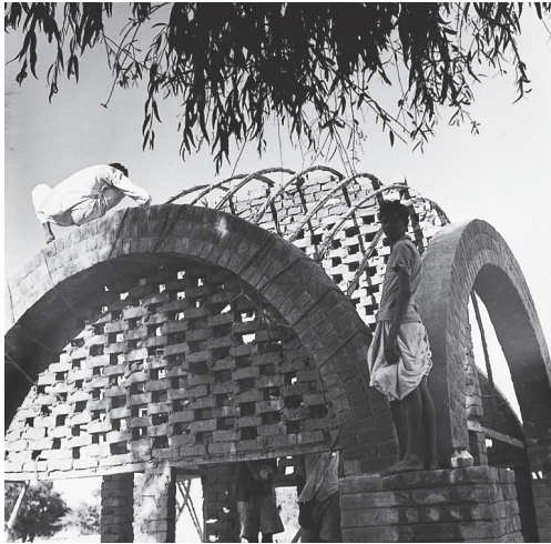
Formwork in place
