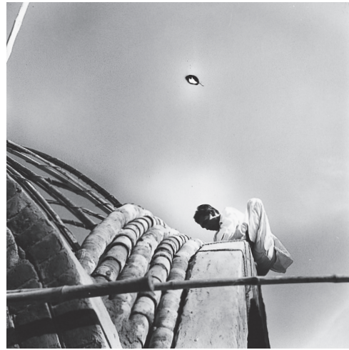
Placing the guna-tile ribs
