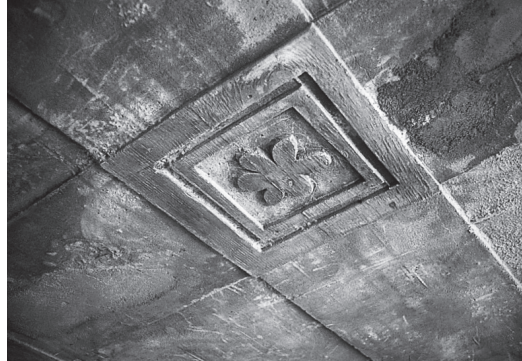
Left: After the gunite shoot. Right: Ceiling detail, in a ceiling formed by gunite shot over cheap styrofoam fillers on a plywood form.
