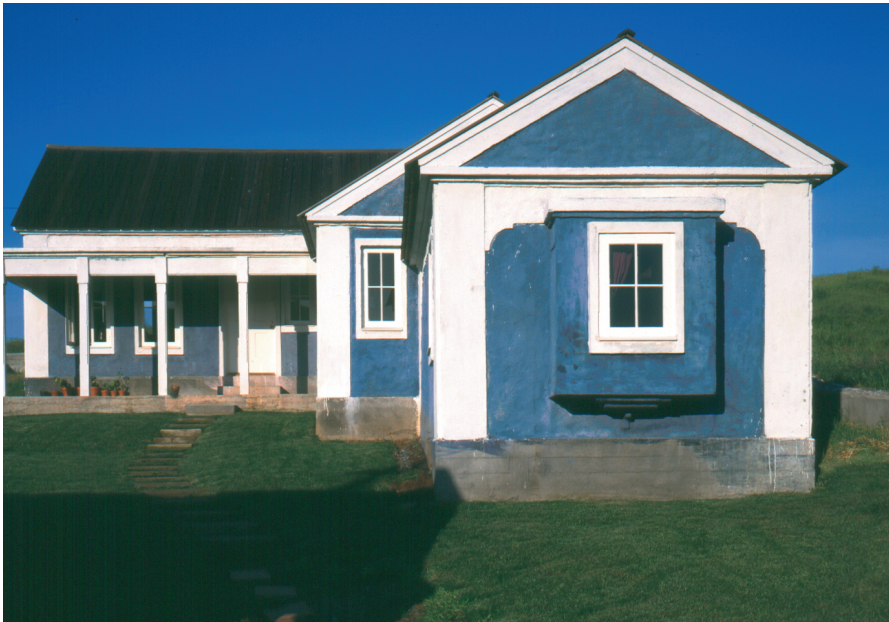
The Martinez gunite house, finished and painted. Christopher Alexander and others, 1978–84.
