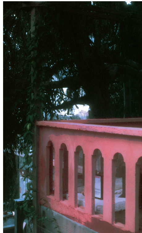
Left: Diagram of formwork. Right: Concrete balustrade made from this kind of form by pouring concrete into low-budget assembly of two sheets of sheetrock, braced, and with hand-cut styrofoam fillers.
