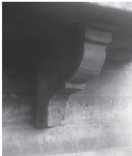
Finished concrete bracket
