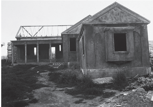
Left: After the gunite shoot. Right: Ceiling detail, in a ceiling formed by gunite shot over cheap styrofoam fillers on a plywood form.
