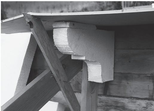
Checking the shape in styrofoam mockup
