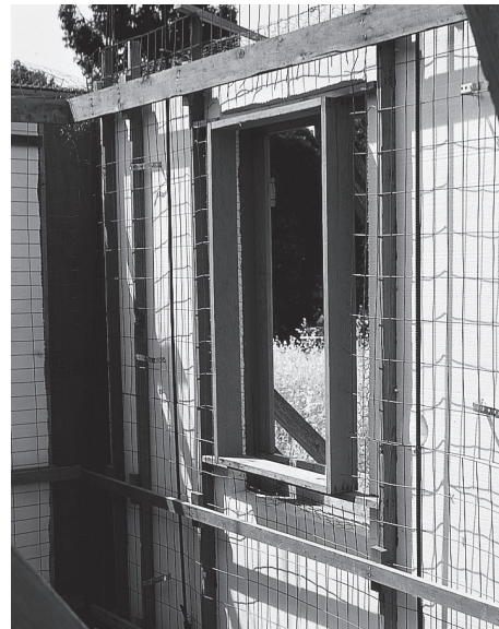
Guidework with mesh and window opening in place
