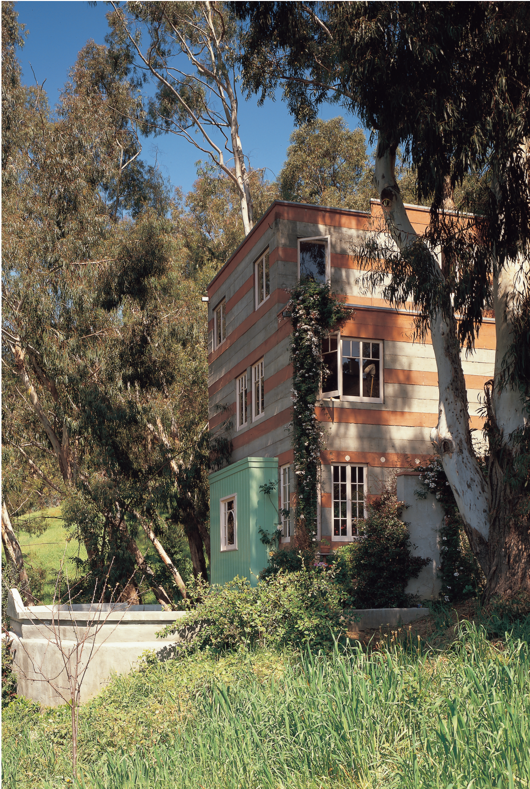
The Sala house, with exterior two-inch concrete shell.
