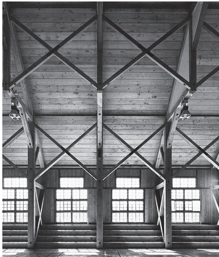
Longitudinal X-bracing inside the gymnasium
