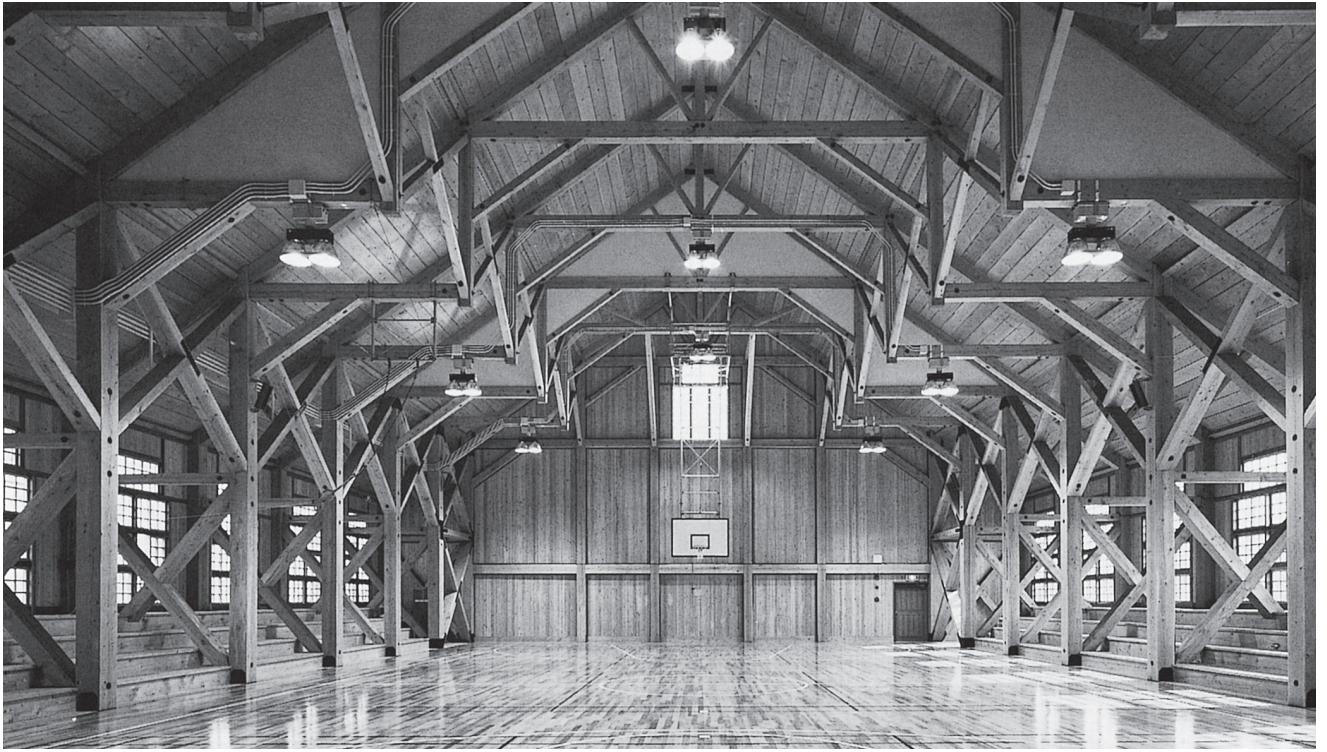
The largest wooden building built in Japan during the second half of the 20th century. The gymnasium of the Eishin school, heavy timber trusses.
