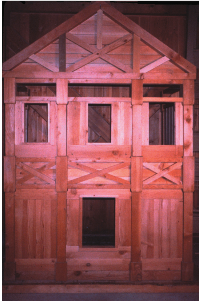
A one-third full-size timber model of a low-cost heavy timber house of 800 square feet that we built and were experimenting with in my office. Here the plastic qualities of heavy timber as a material that can be shaped and carved, become clearly visible. The whole house is built as a three-dimensional truss, with a lifetime of many centuries: easily justifying the use of heavy timber as both cost-effective and sustainable. Christopher Alexander, 1986.
