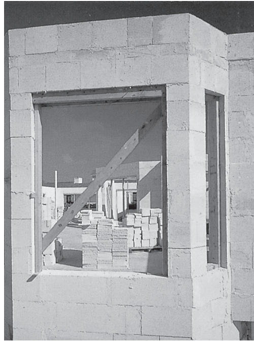
Lightweight Hebel blocks which can be hand cut and shaped with woodworking tools, being used in construction of a small factory.
