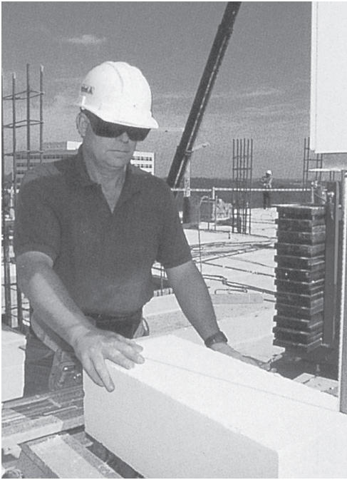
Lightweight Hebel blocks which can be hand cut and shaped with woodworking tools, being used in construction of a small factory.
