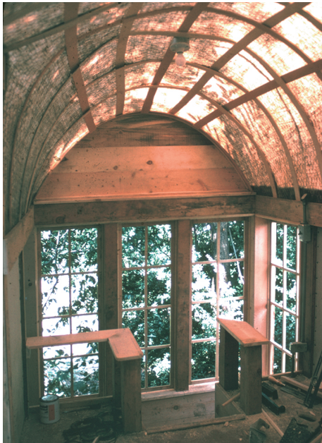
Interior of the Etna Street cottage, Berkeley, 1973. Left: Burlap impregnated with fiberglass resin forming a translucent roof. Right: Alcove under the stair, made with a lightweight concrete vault.
