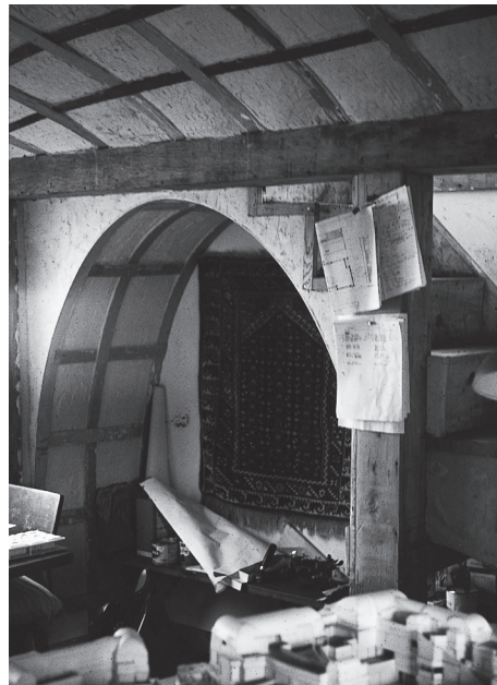
Interior of the Etna Street cottage, Berkeley, 1973. Left: Burlap impregnated with fiberglass resin forming a translucent roof. Right: Alcove under the stair, made with a lightweight concrete vault.
