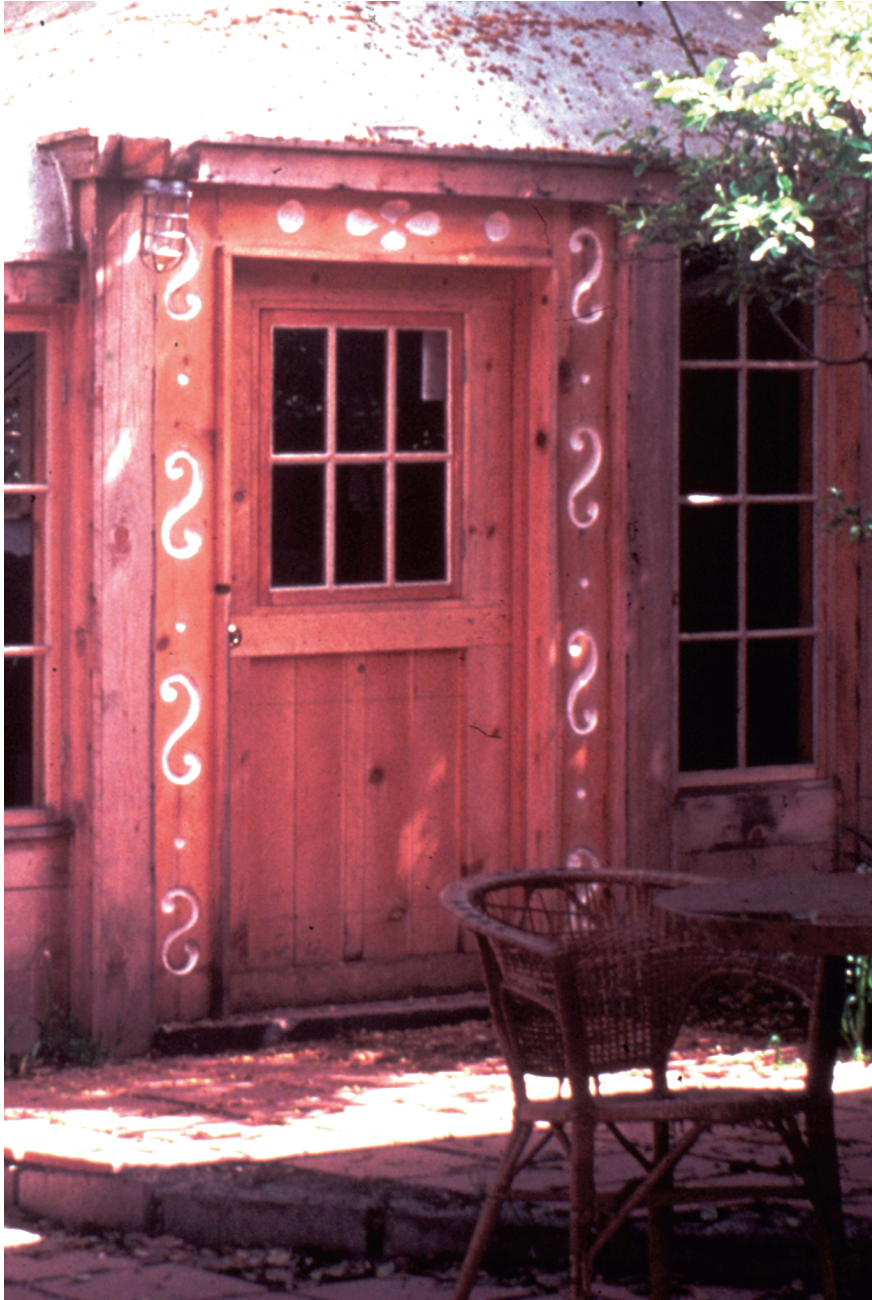
Ornaments which I cut with a jigsaw into the doorframe of the Etna Street cottage, and then filled with plaster, 1973. The ornament came into my mind directly while building the door-frame. With a pencil and a jigsaw, and then with a few trowels of white plaster, the whole thing was done. It came directly from the whole, was inspired by the whole, and then activated and made accordingly.
