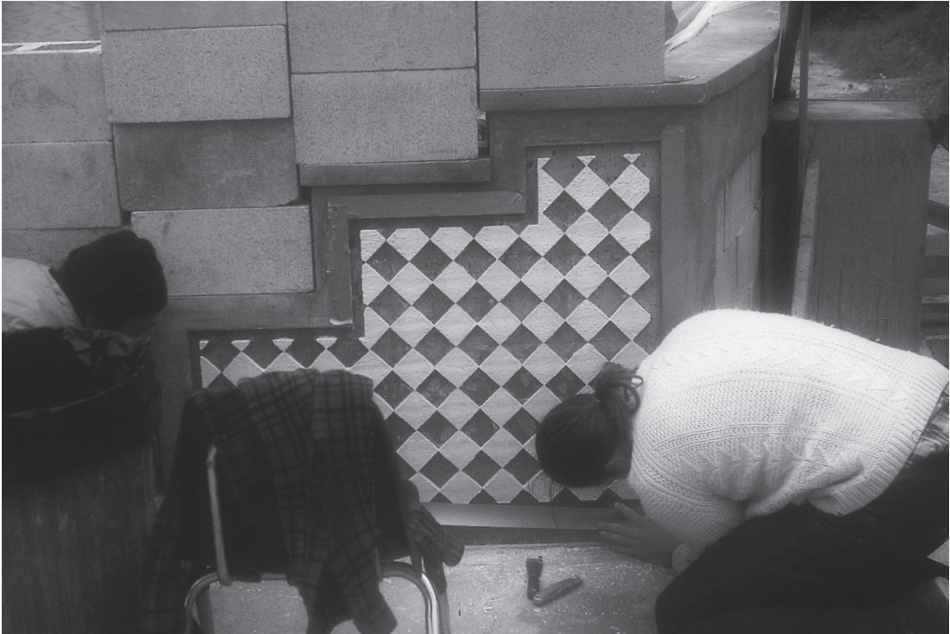
Correction of details in the formwork
