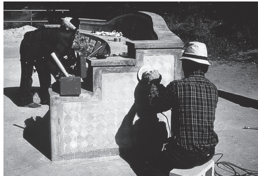
Grinding after completion of wet phase
