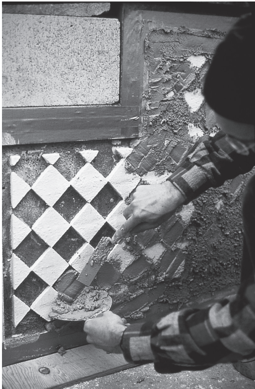
Placing marble-cement mix into the formwork
