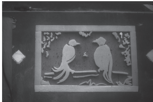
Formwork of another ornamental panel, Fort Mason bench.
