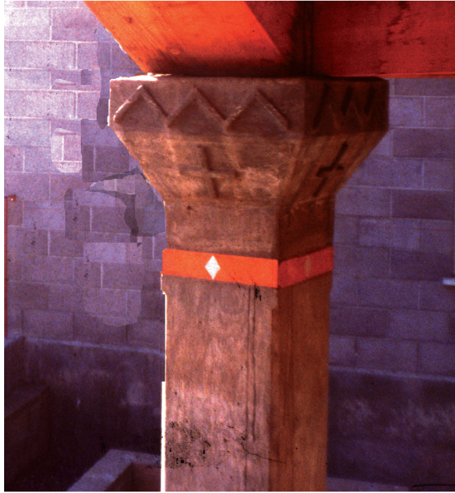
Ornamental detail of a cast column capital for the Julian Street Inn, California. Christopher Alexander and Steve Murray, 1989.
