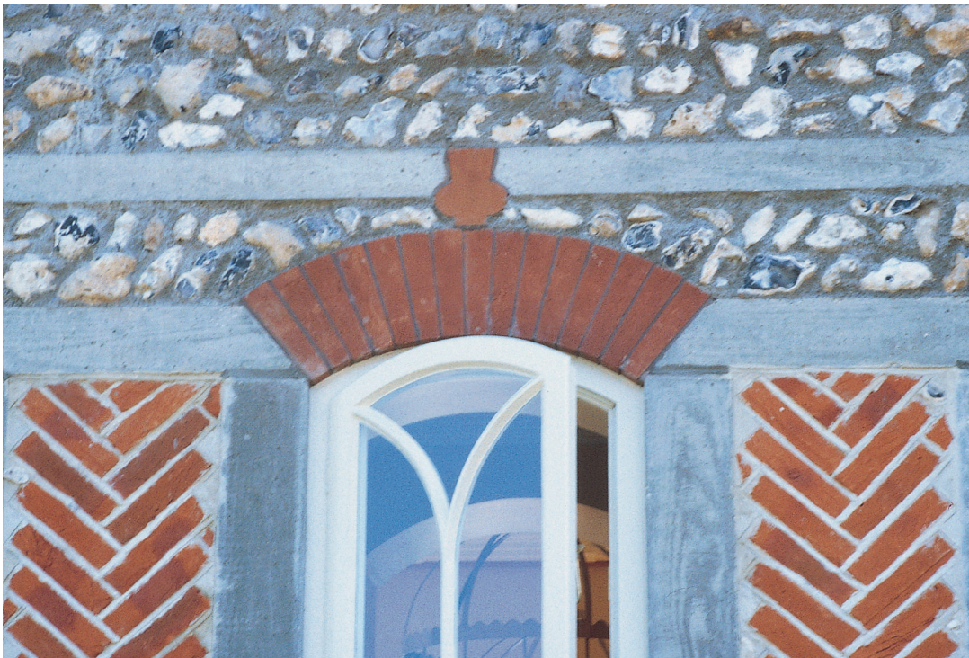
Brick pattern, arch, window muntins, and thistle ornament at West Dean. Christopher Alexander and John Hewitt, 1995
