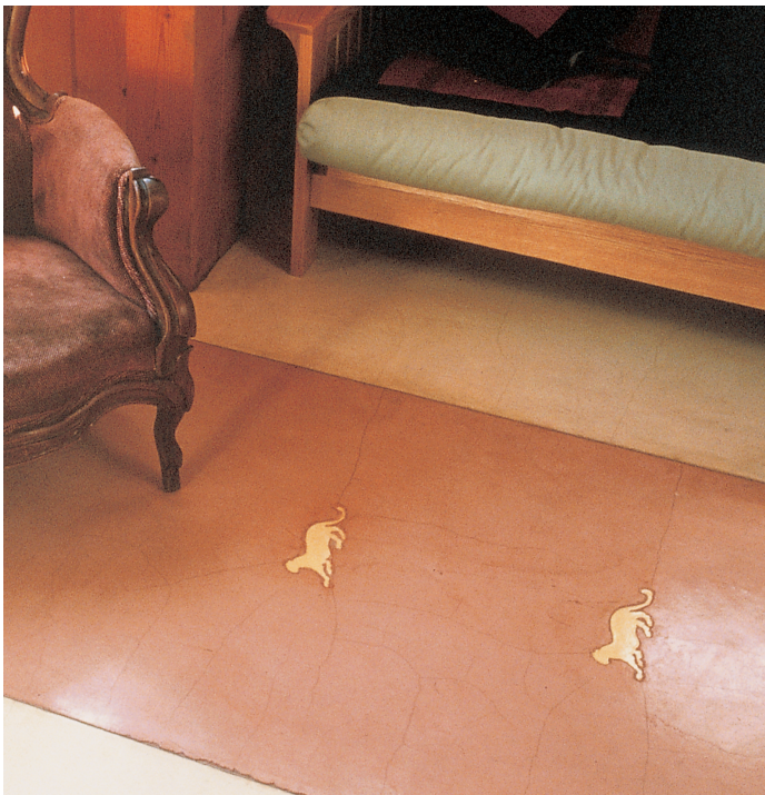
Ceramic leopards I placed in concrete floor of the Sala's second house.
