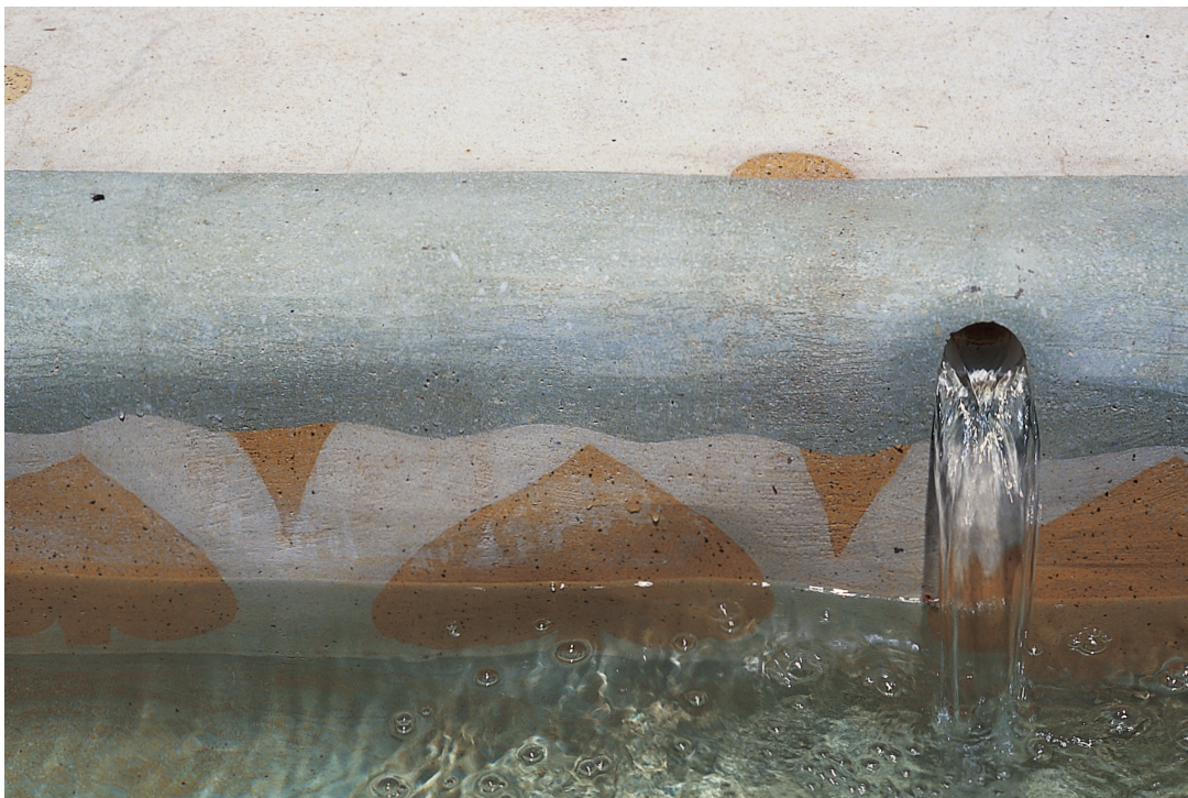
Green and yellow terrazzo, as we built it in the Sarlo tubs. Christopher Alexander and Eleni Coromvli, 1986.
