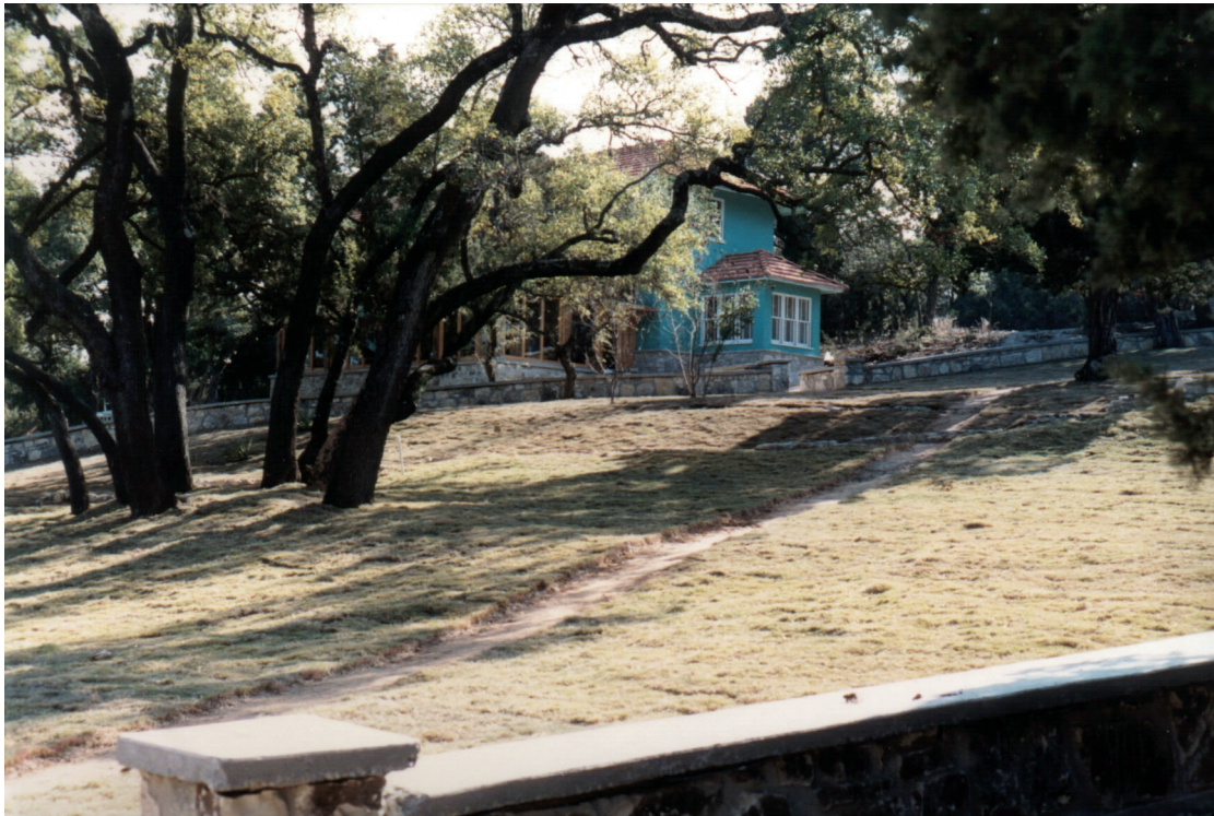
The core of public space, as it appeared when finished, with the individual houses all around it. Back of the Moon, Austin, Texas. Christopher Alexander, Saul Picardo, Randy Schmidt, 1995.
