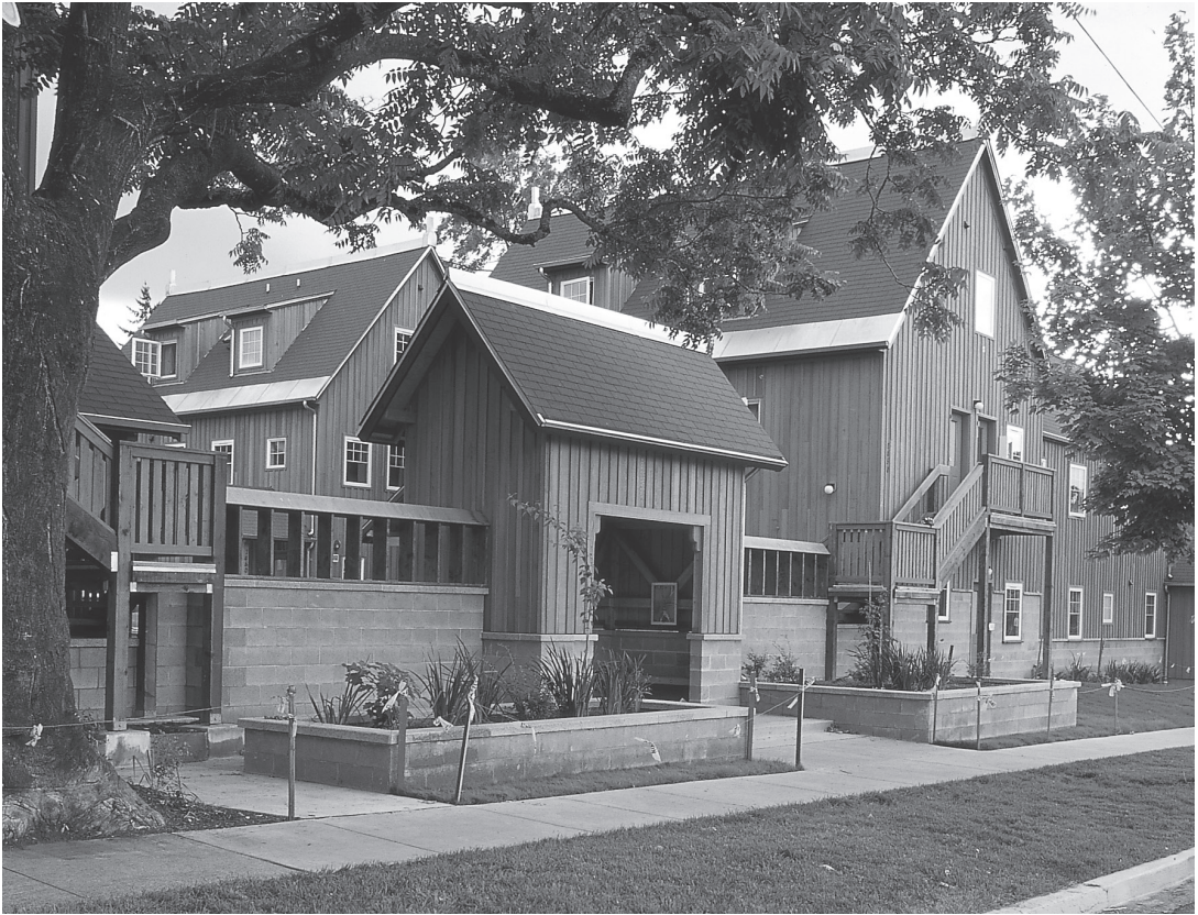
The entrance gate from the street to a very small domain of public space, a public hull in miniature. Agate Housing, Eugene Oregon; Christopher Alexander, Hajo Neis, James Maguire and others, 1992.
