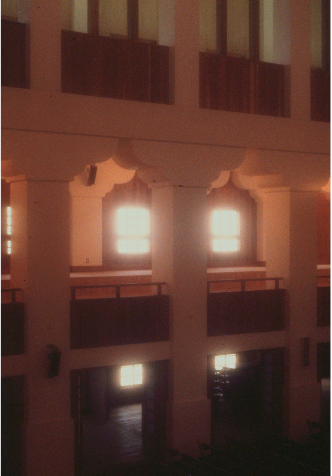
Luminous plaster on the interior columns and capitals of the Great Hall, Iruma-sbi, Tokyo, first state of completion. Christopher Alexander, Ingrid King, Hajo Neis and others, 1985.
