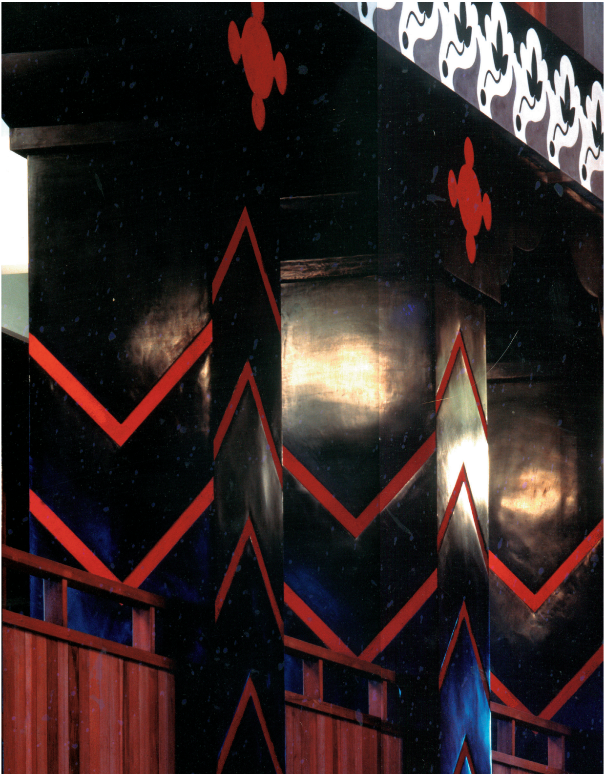
Columns of the Great Hall. The mirror surface of the columns is polished black plaster known as Shikkui, an ancient Japanese technique (Book 4 page 47 and Book 2 pages 378–83). If you look at the black space between two red chevrons on the face of the leftmost column, you see that this black space is a living center, which is itself composed of two black rhombuses leaning away from each other, themselves also living centers. There are living centers everywhere.
