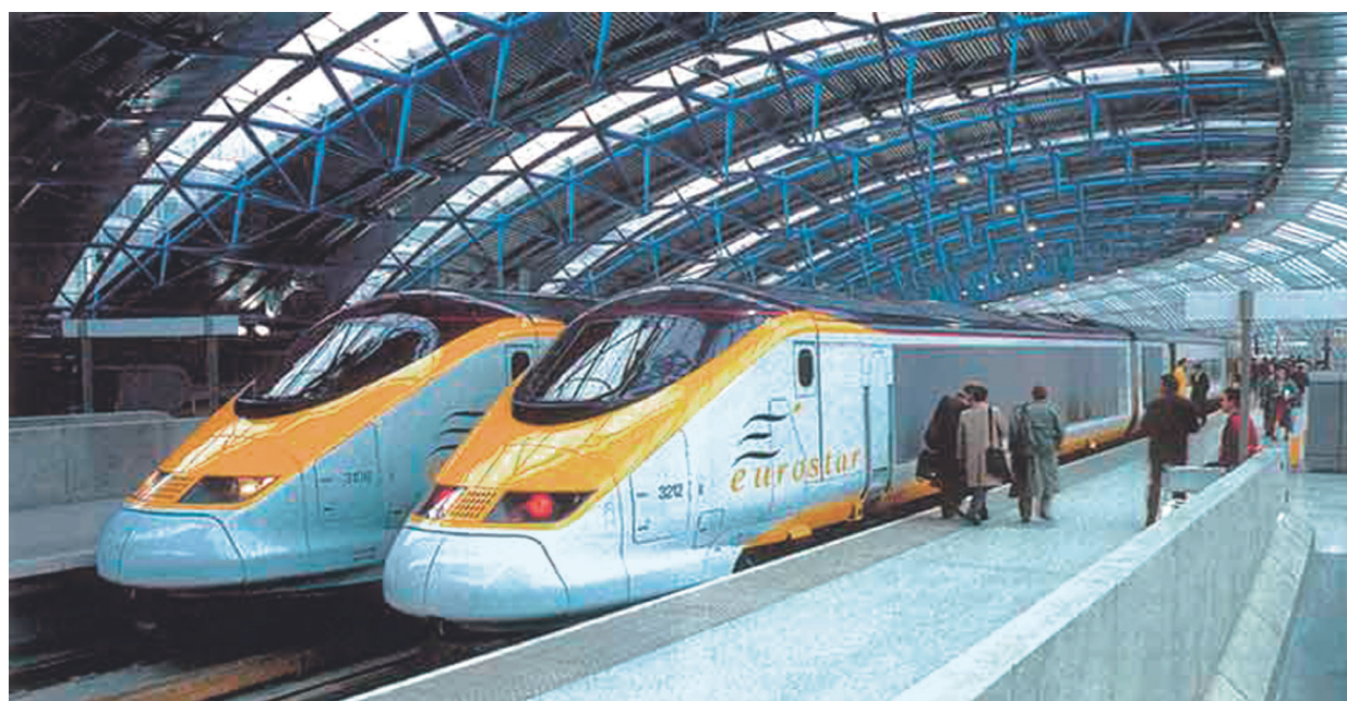
The Eurostar Terminal, Waterloo, London. Architectural design Nicholas Grimshaw, engineering design Anthony Hunt, 1993
