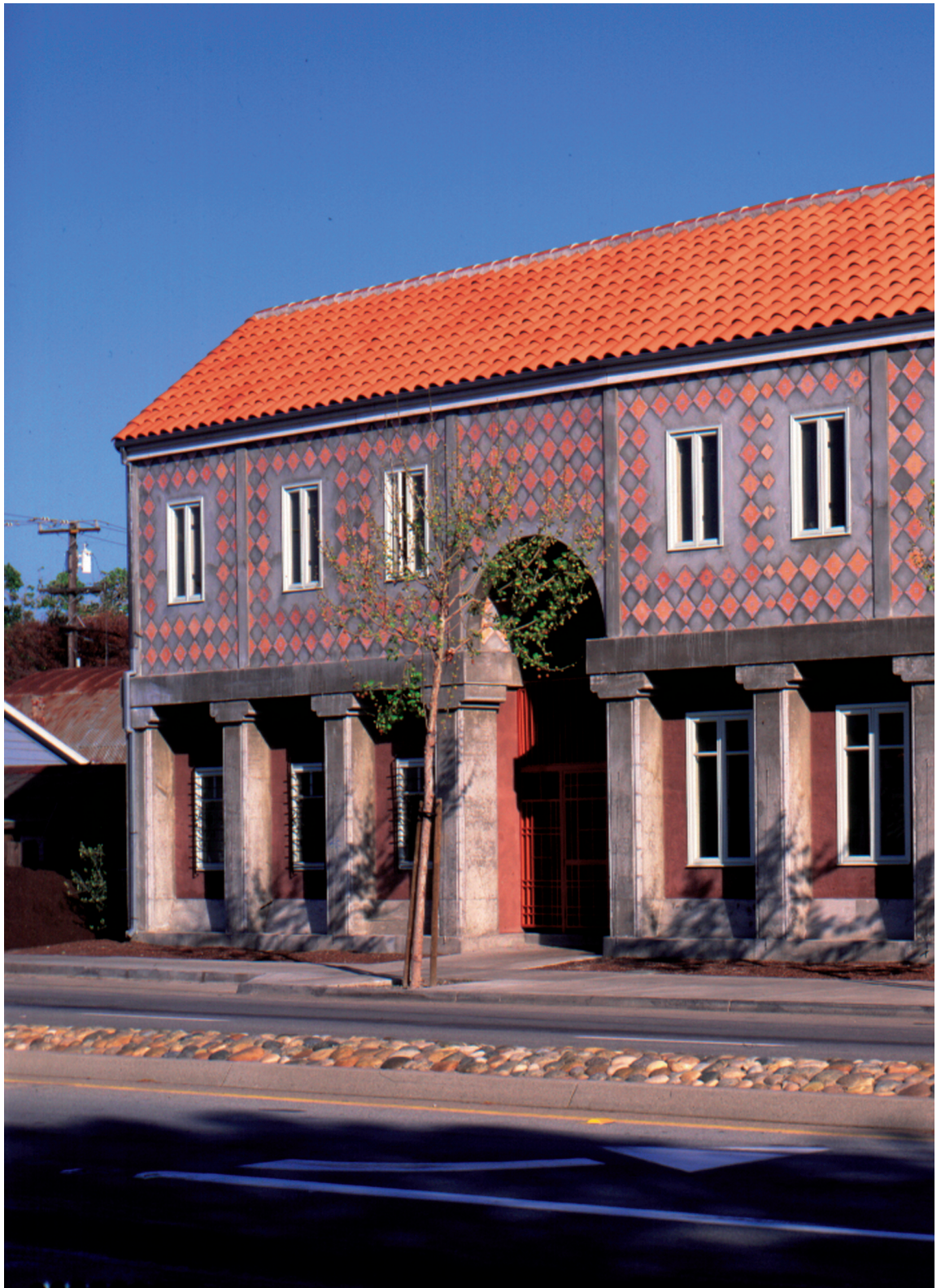
Note the hand-painted tiles on the upper wall surface. Four thousand of these tiles were made for the building in our own workshops. See extensive discussion about the tiles in Book 2, pages 292–95.
