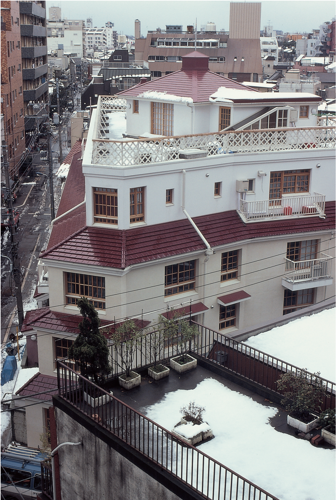
The Emoto apartment building, Tokyo, Christopher Alexander with Hajo Neis, Ingrid King, Miyoko Tsutsui, 1987
