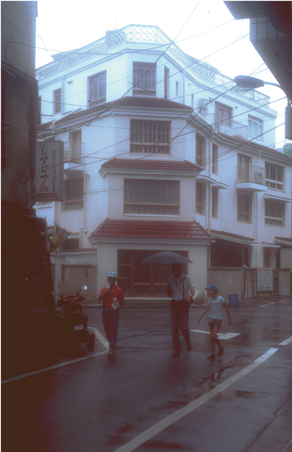
A rainy day in Tokyo: The completed Emoto apartment building, Christopher Alexander, Hajo Neis, Ingrid King, Miyoko Tsutsui, 1987.
