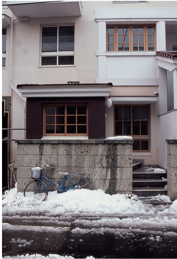
Winter 1988. An exterior, street-level view of one apartment in the Emoto building. The simple, nearly stark, but comfortable, solid quality of the building comes from the unfolding—especially from the inclusion of NOTHING extra BEYOND the decisions of unfolding.
