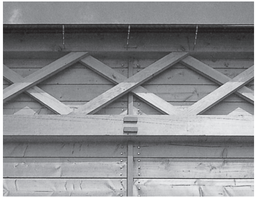
X-braces of the Central building, showing the POSITIVE SPACE between the wooden members.
