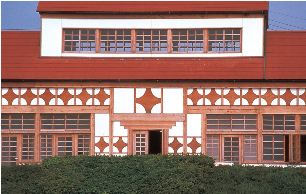
Structural frame of the Cafeteria building, Eishin campus. Christopher Alexander, Hajo Neis, Gary Black, 1985
