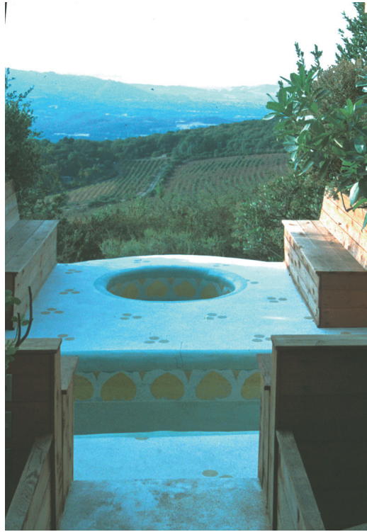
Hot and cold tubs overlooking vineyards of the California hills, hand-ground colored marble dust, Sonoma, California. Christopher Alexander, Eleni Coromvli and Mark Briner, 1985
