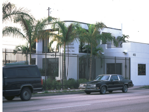
A recently built business in Progresso. It fits in to its environment. It is helpful, pleasant. It has the right scale and, with its garden of palms trees, helps the community.
