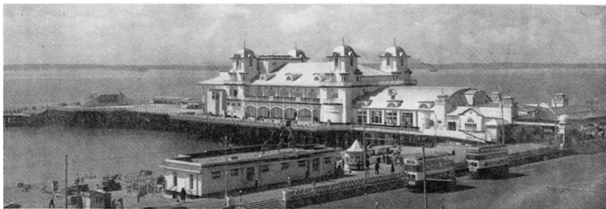
South Parade Pier, Southsea—setting for the Portsmouth Symposium on Design Methods in Architecture, which attracted some 400 delegates, including 50 from overseas
